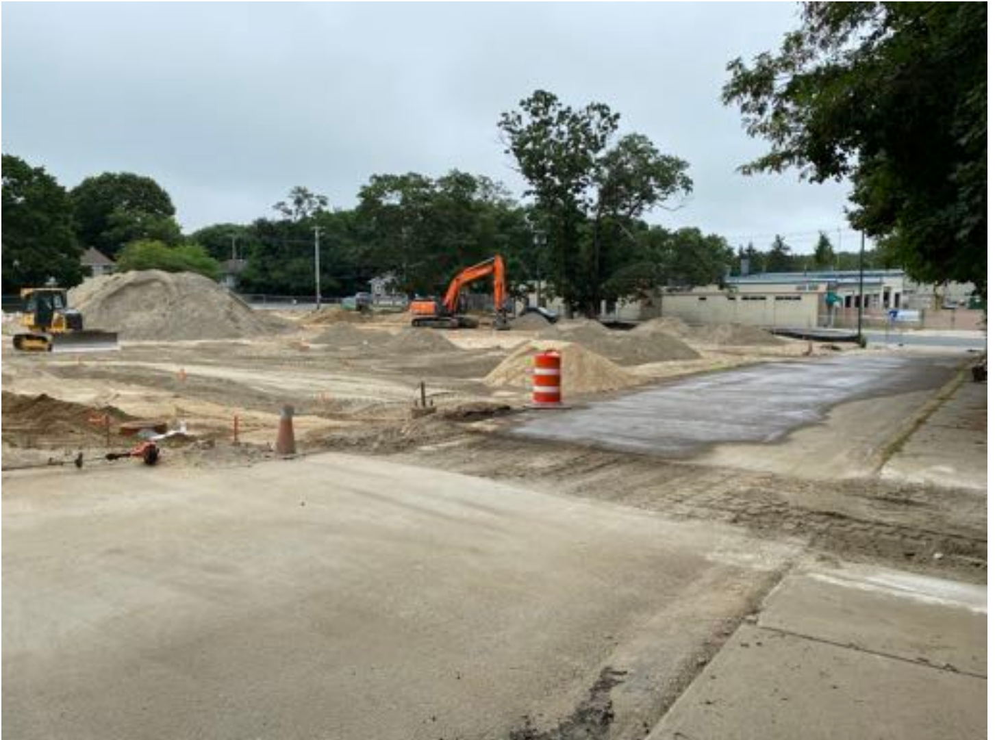
Driveway cleaned before storm
