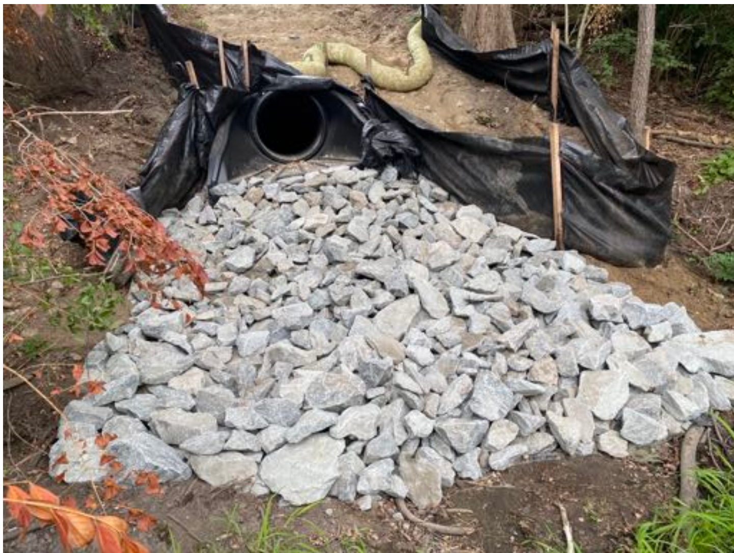
Flared end level spreader installed
