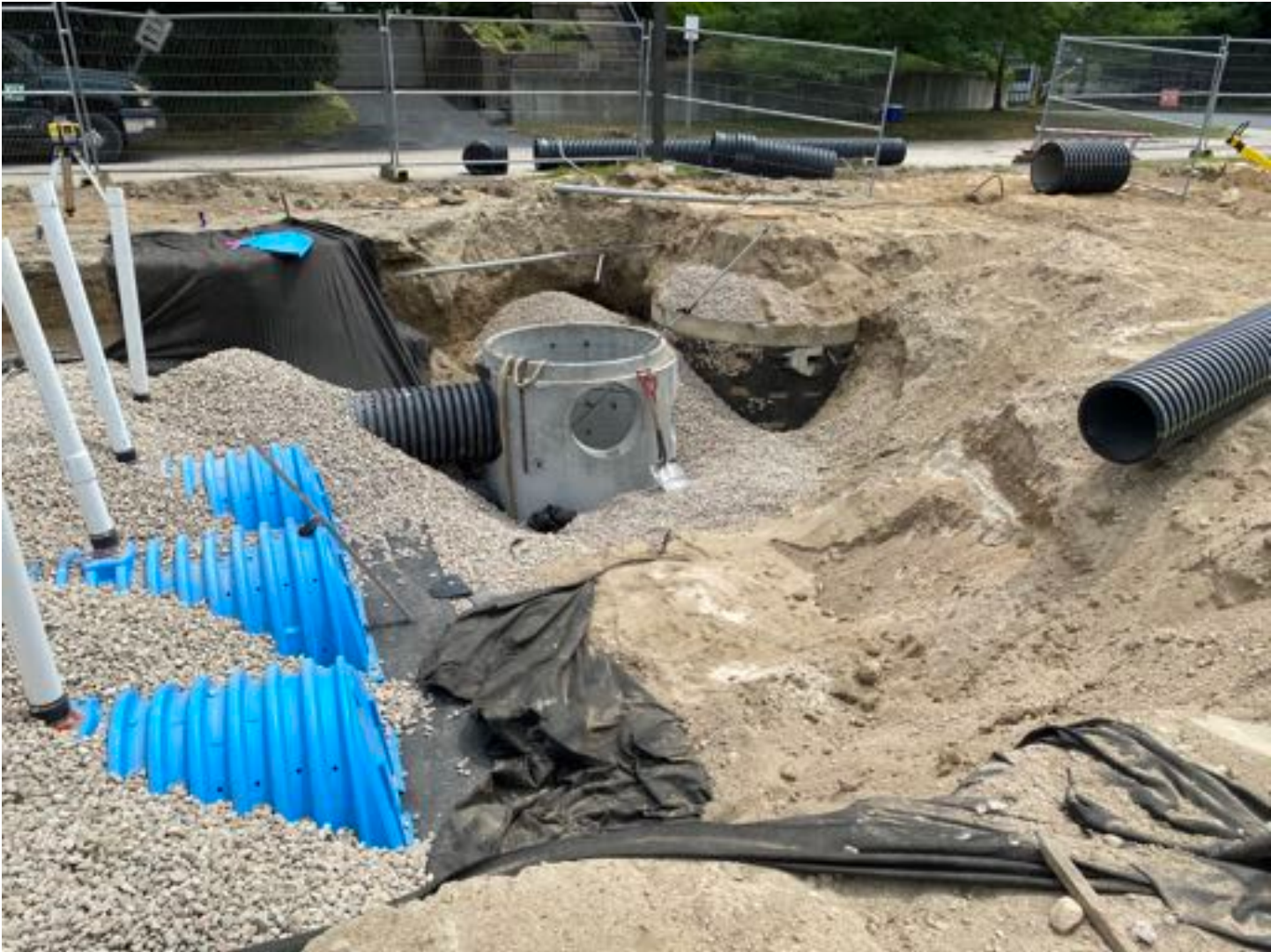
DMH #1 installation
