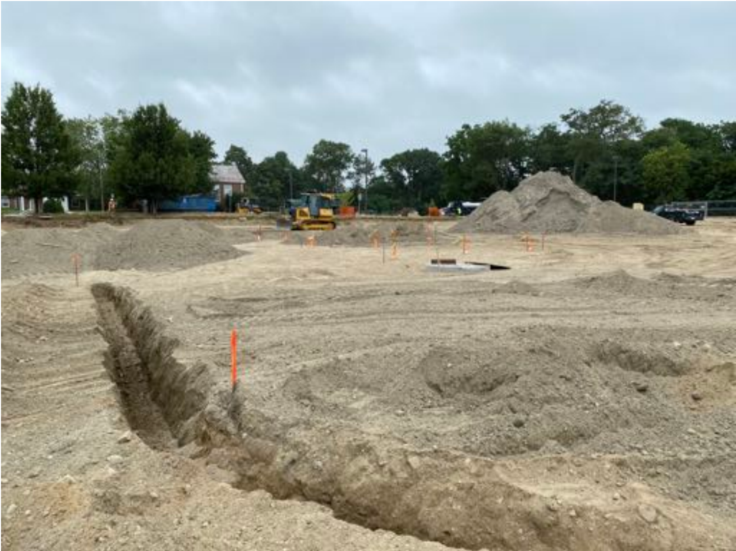
Electrical trenching/UCS clean outs adjusted.
