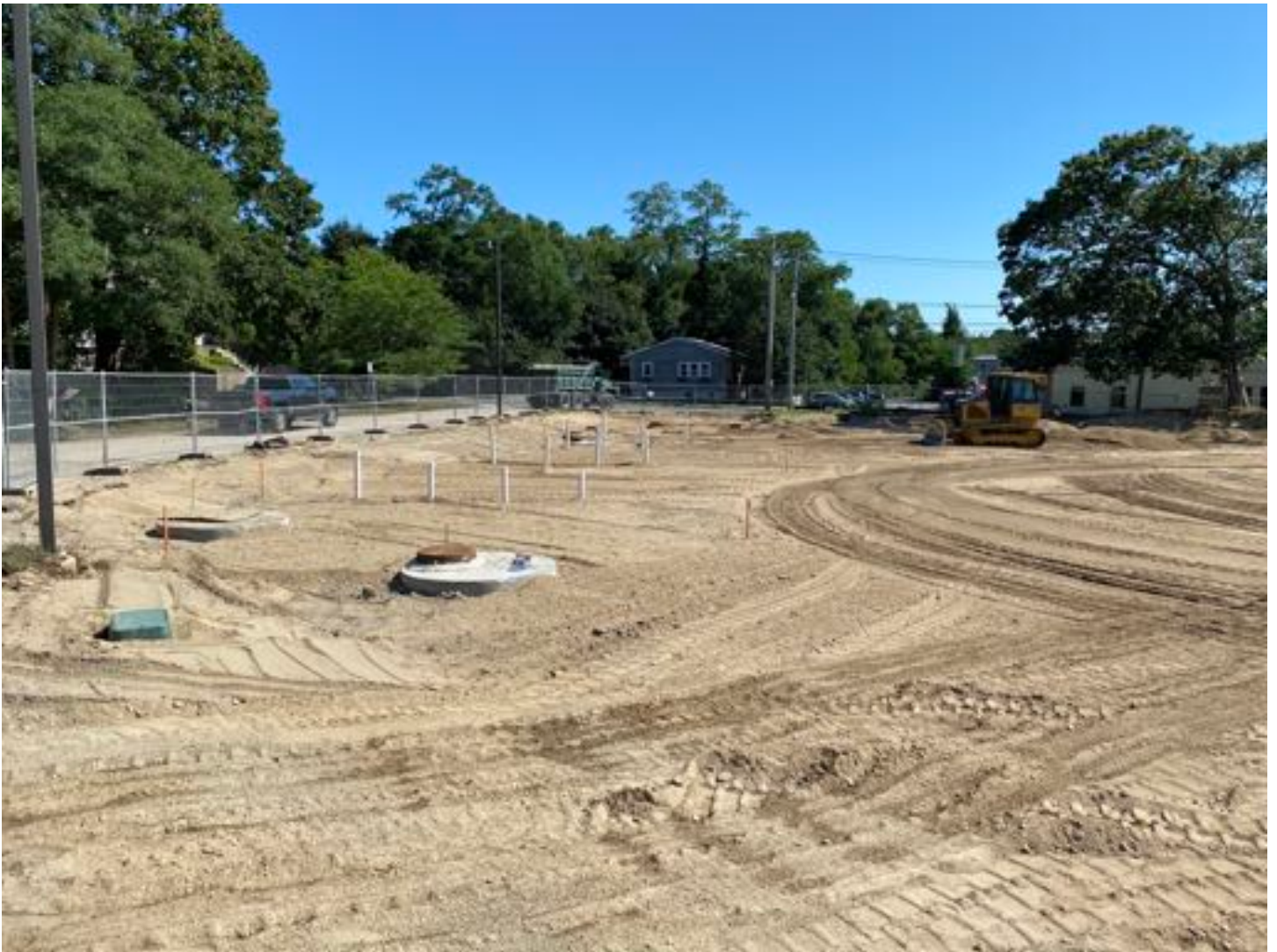
Subgrade prep in eastern half of main parking lot.
