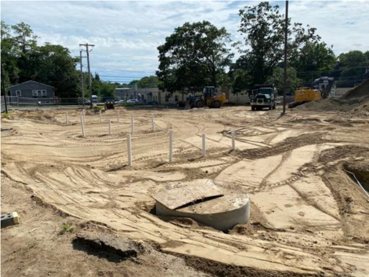
UCS #2 backfilled
