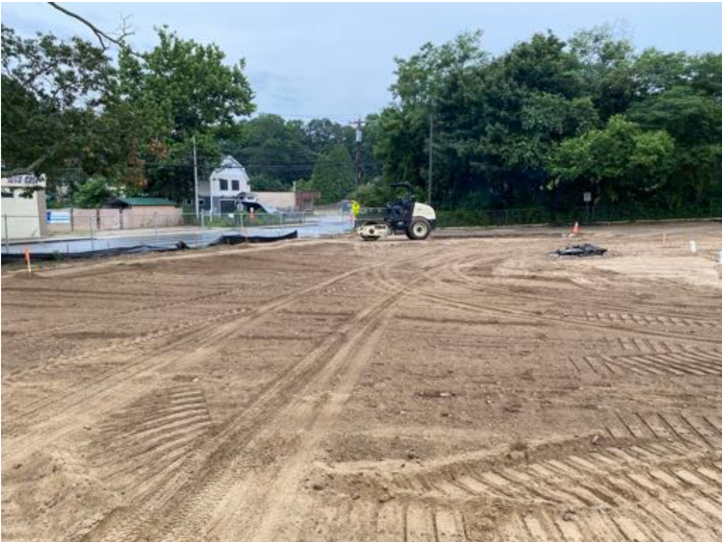
Subgrade prep in southwest corner of main parking lot
