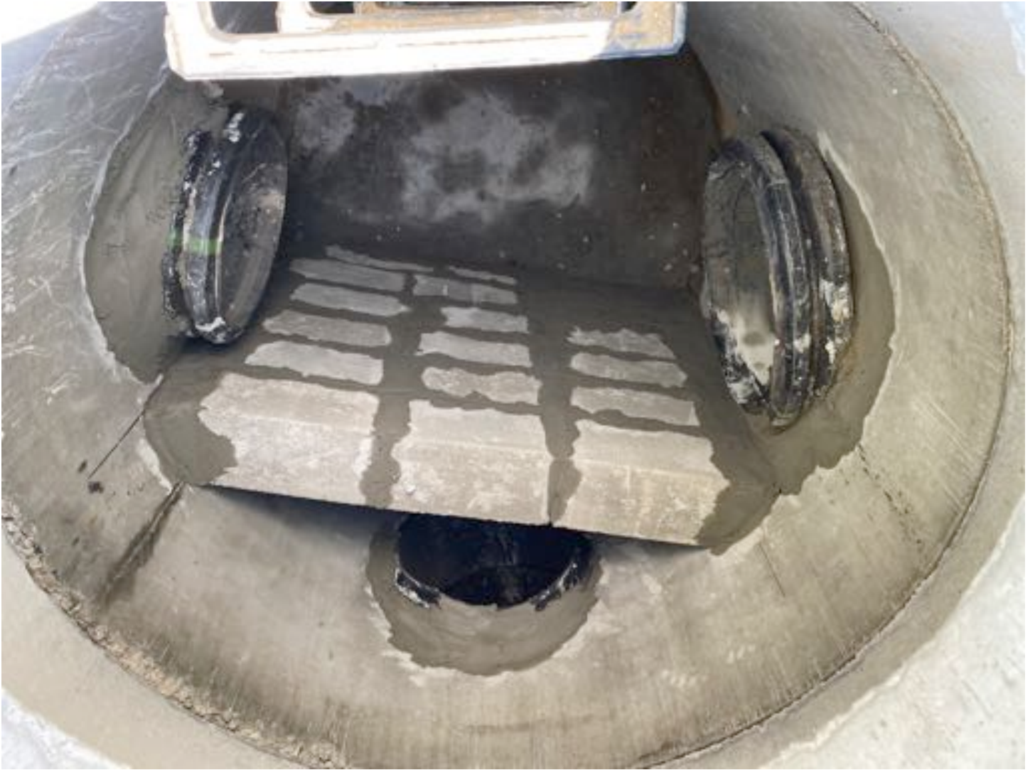
UCS DMH weir installation
