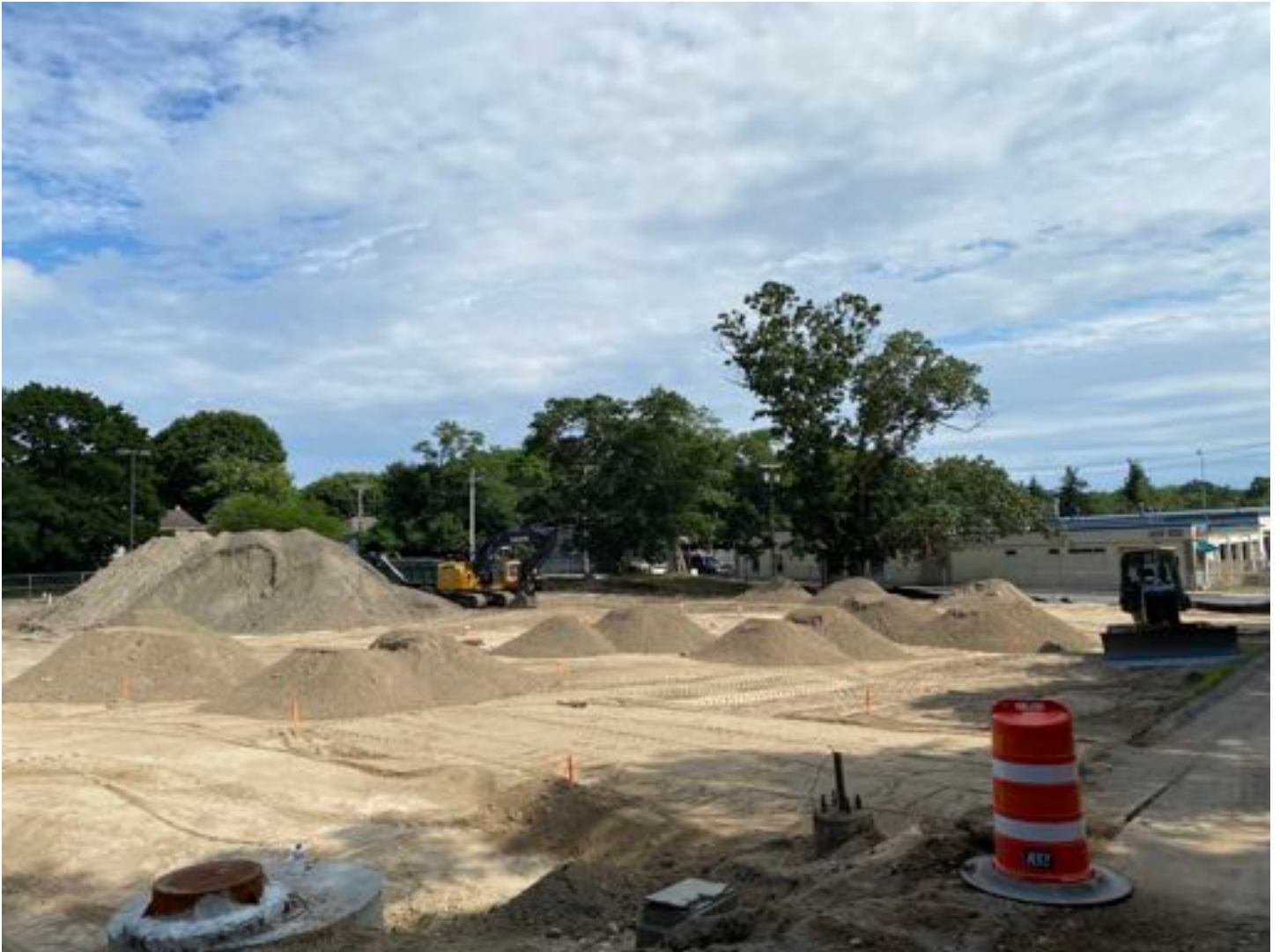
Placement of reclaim base in western half of main parking lot
