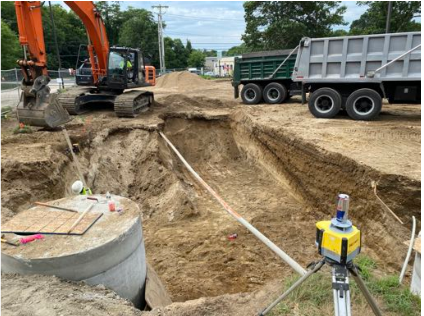
Excavation for UCS#2
