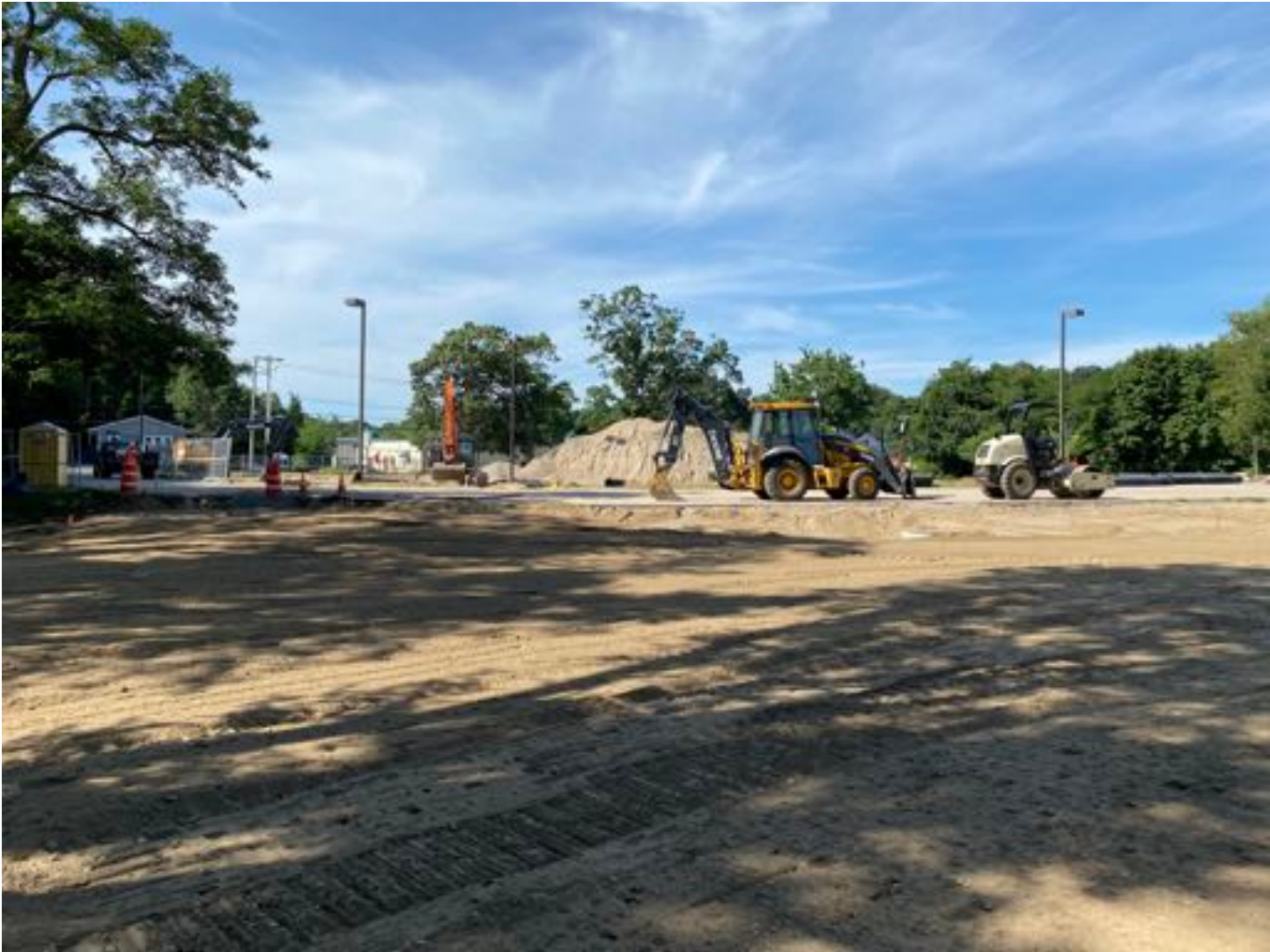
Placement of spoils in expanded parking area complete. Subgrade achieved.
