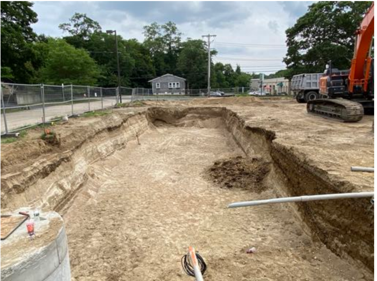
UCS#2 excavation nearly complete.
