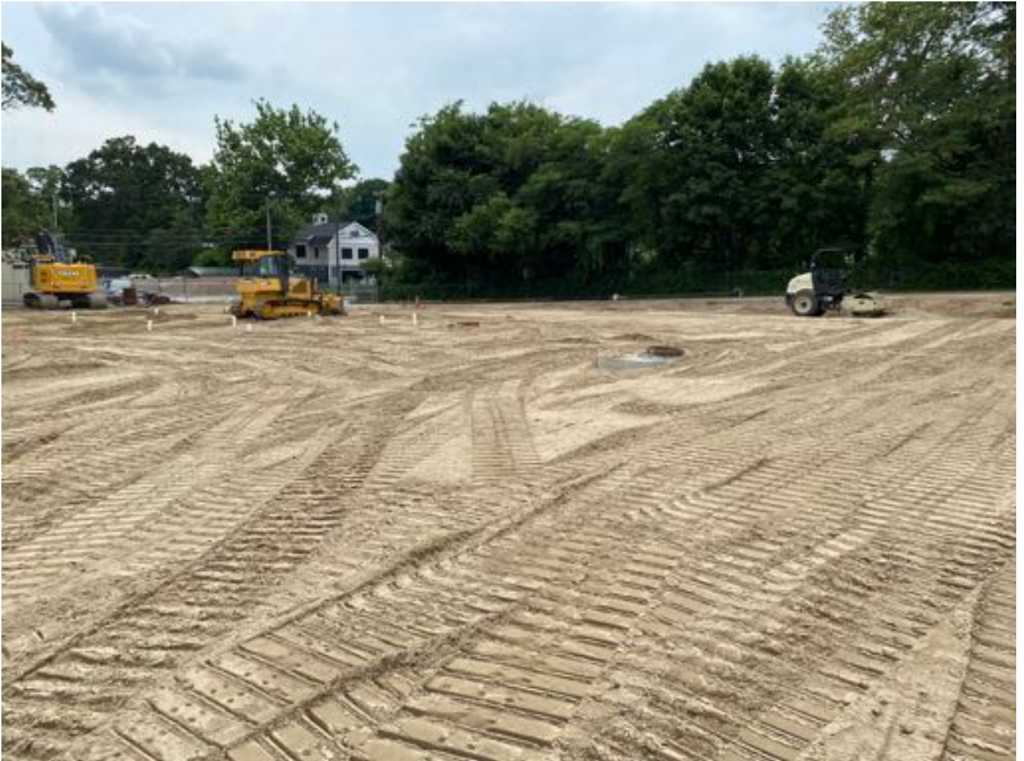
Excavation spoils placed in northwest corner of main parking area.
