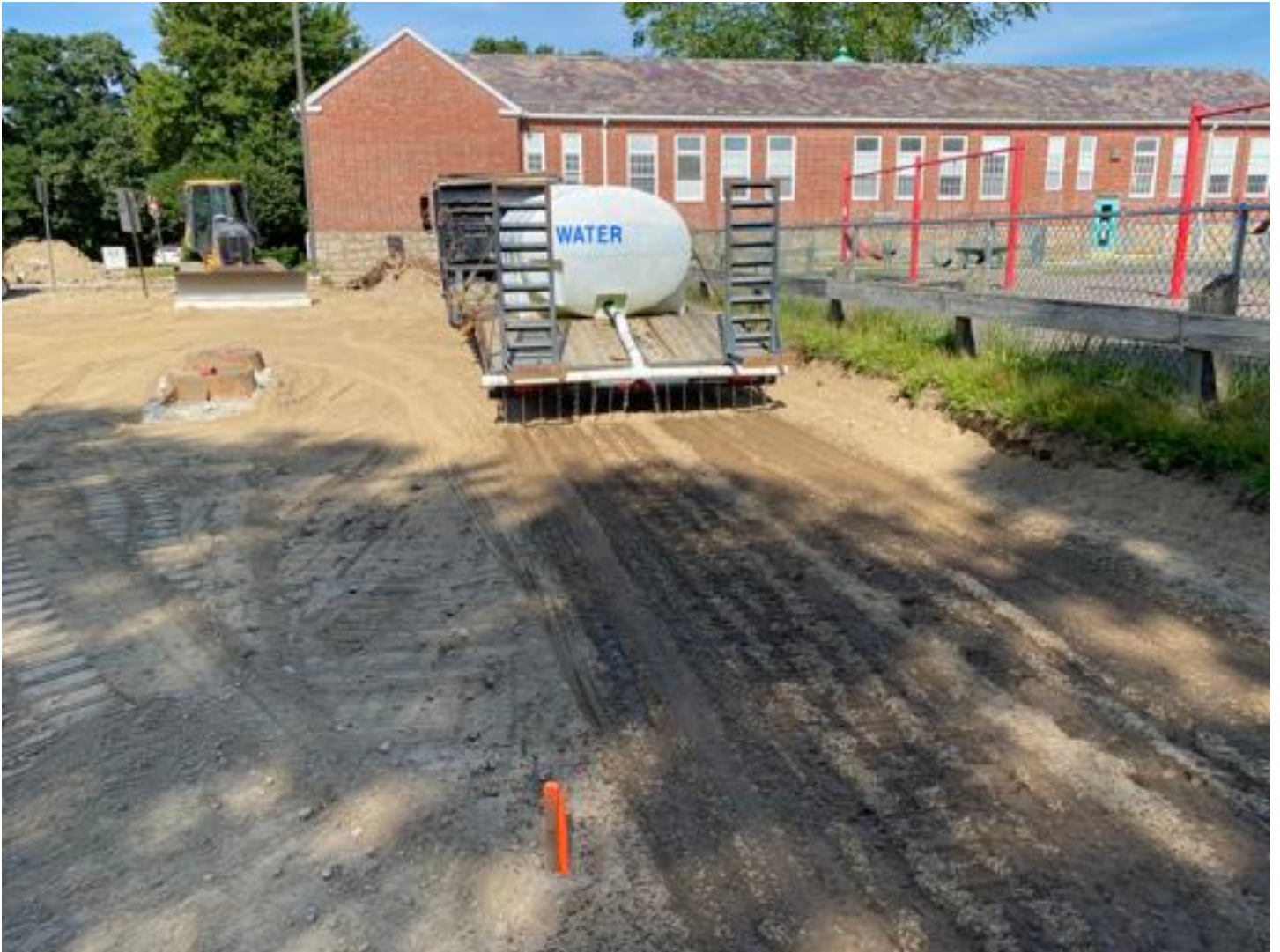
Water placement on dry material before compaction
