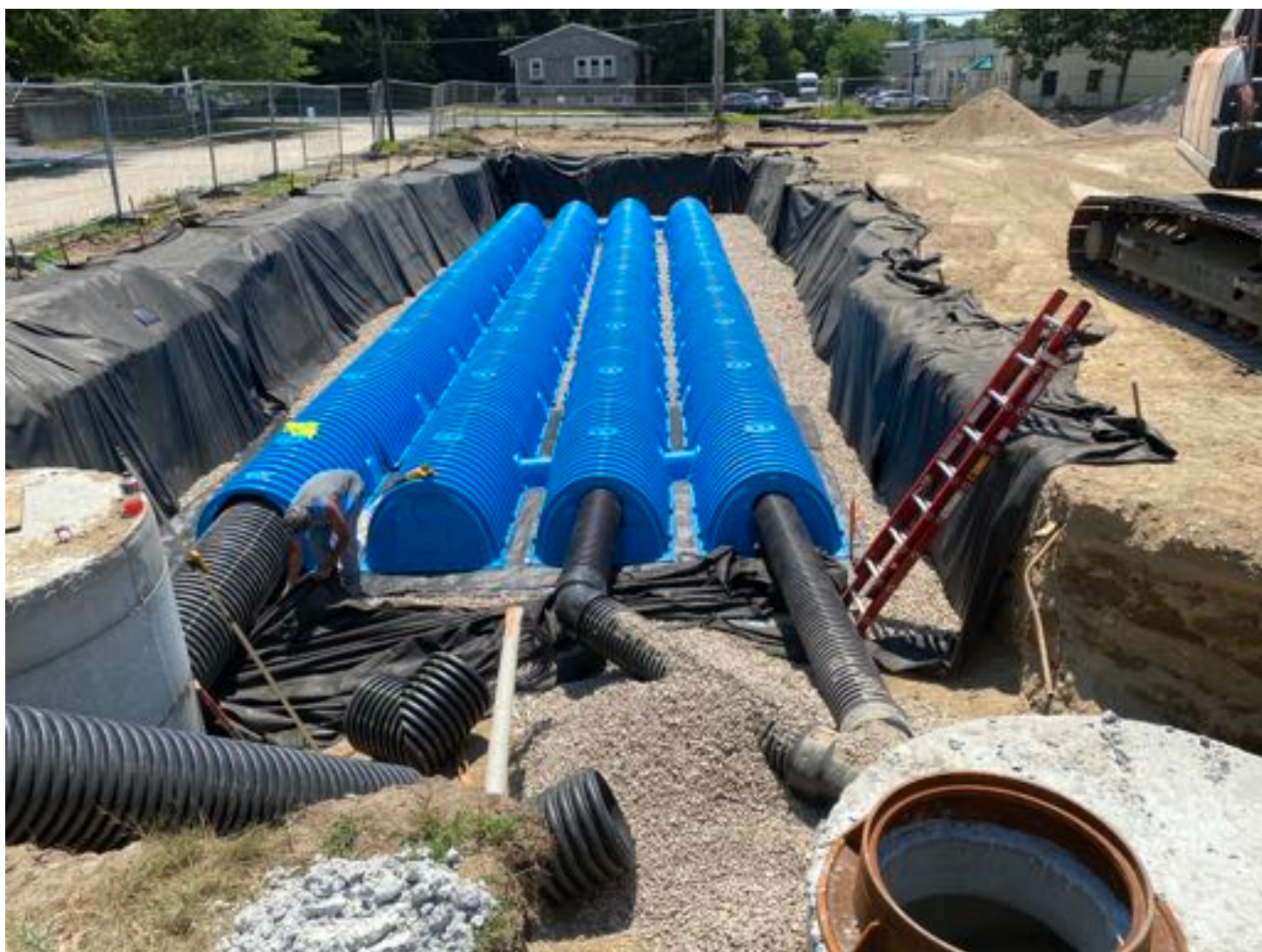
Chambers/pipe placement on north end of UCS #2.
