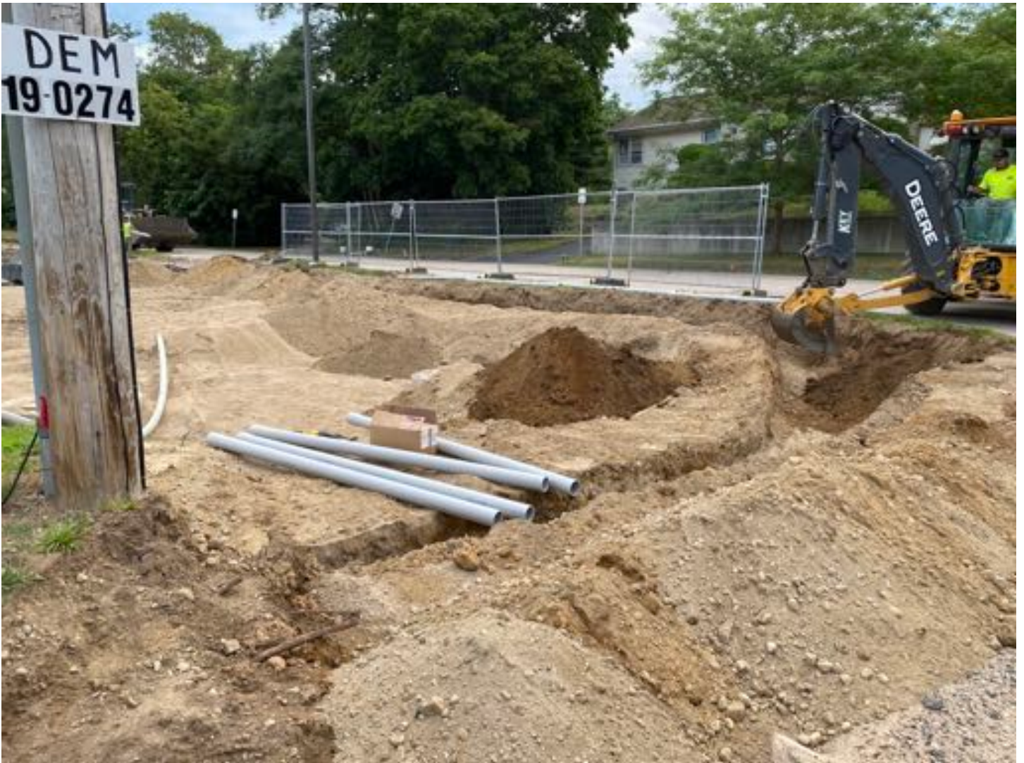
Excavation for COX 4" conduit.
