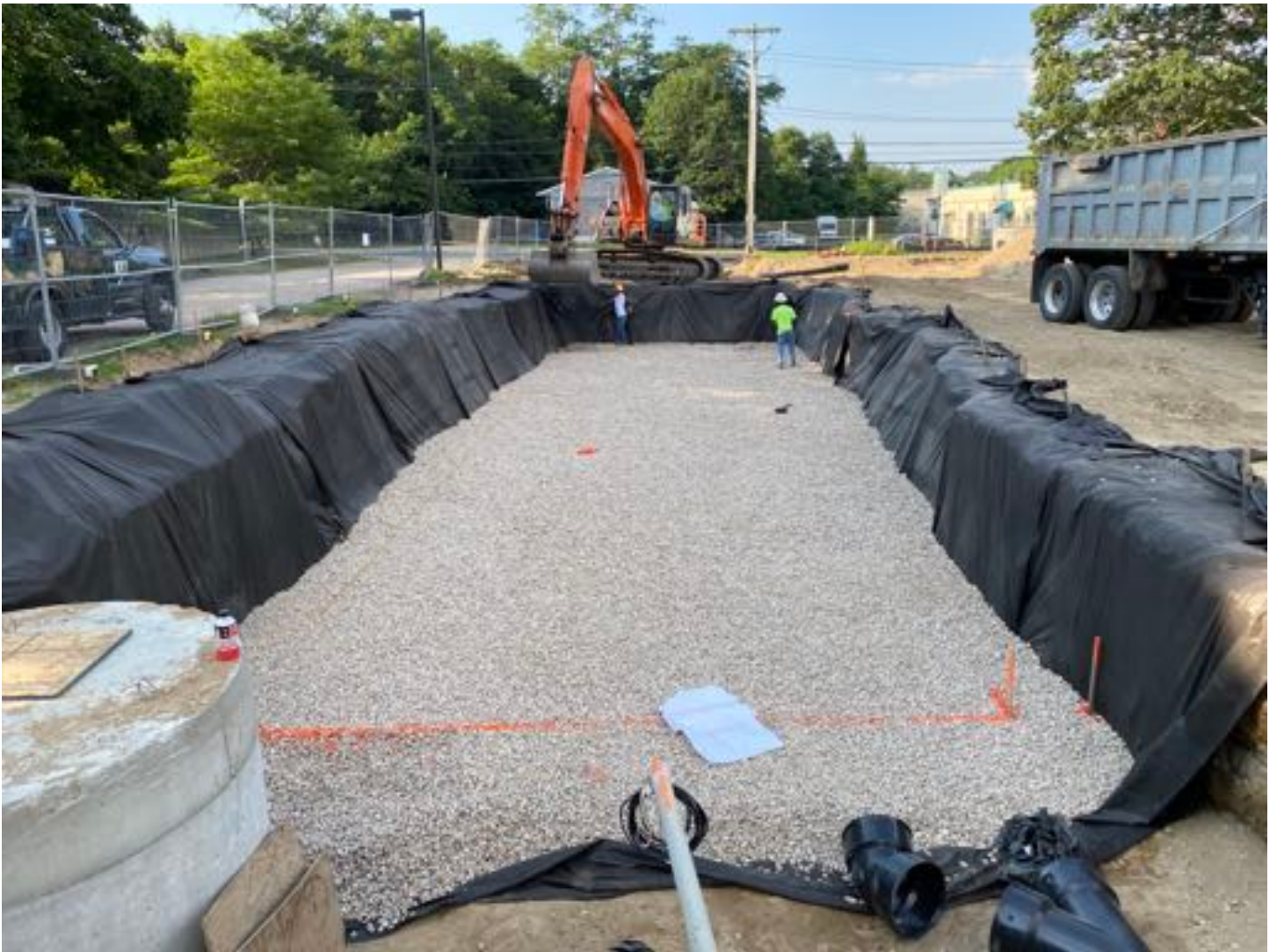
UCS #2 fabric & stone bedding placement complete
