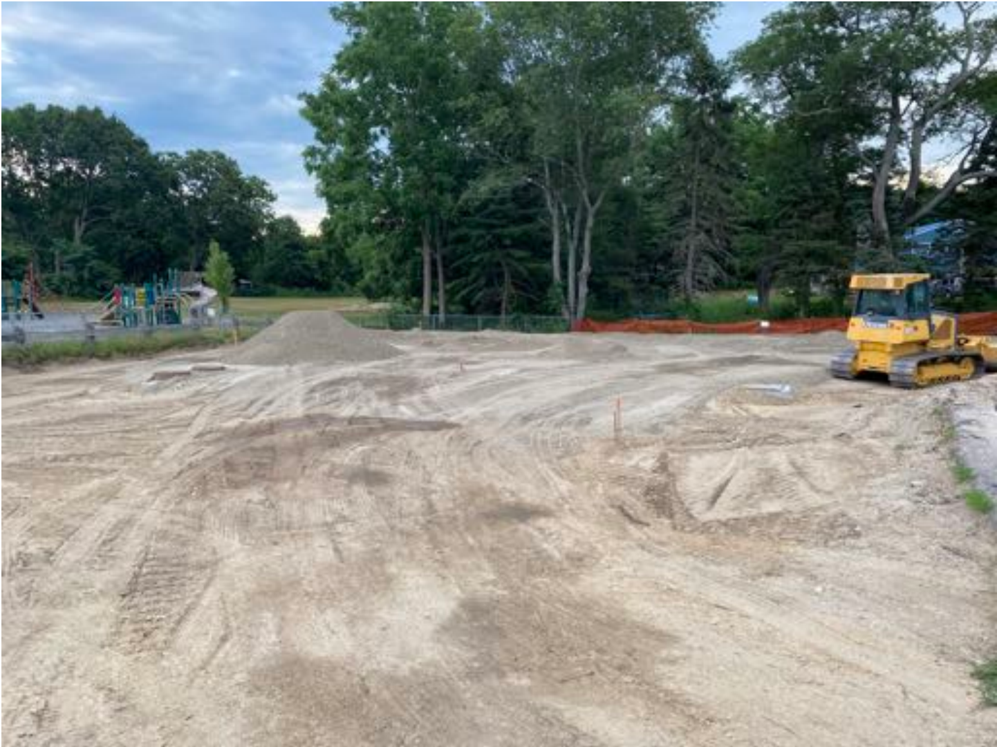
Placement of reclaimed base in expanded parking area.
