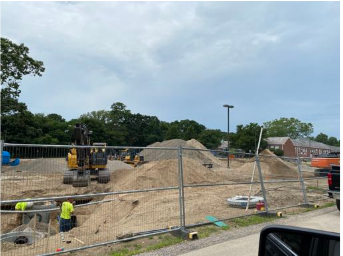
Installing CB's 5 & 6 and associated pipe.
