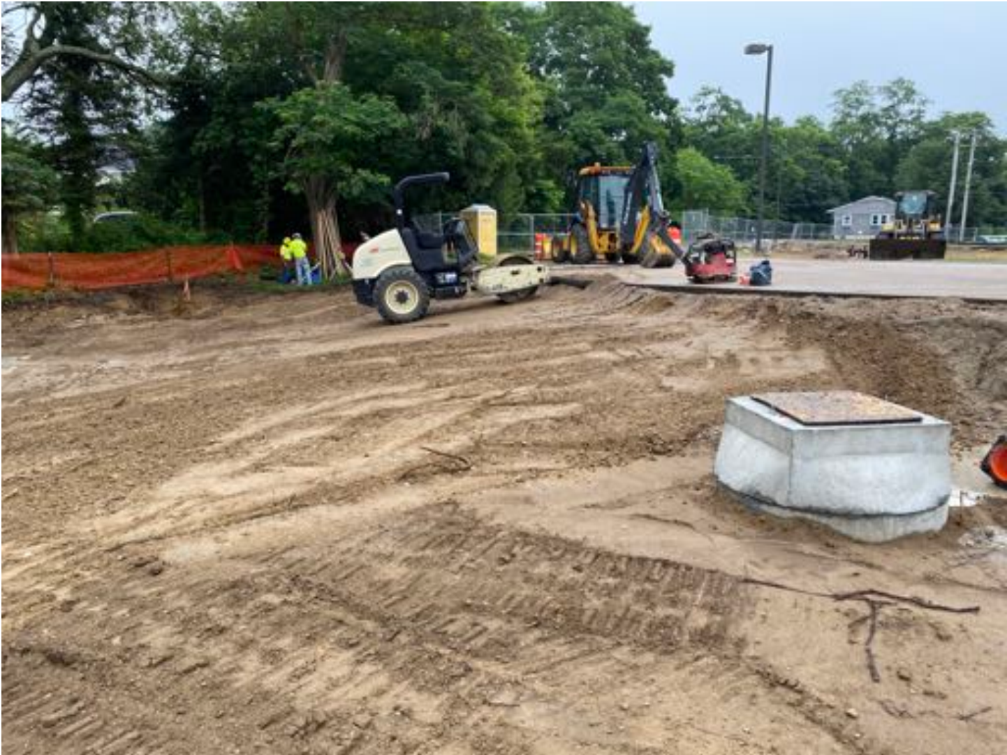
Pipe between CB's 7 & 9 backfilled.
