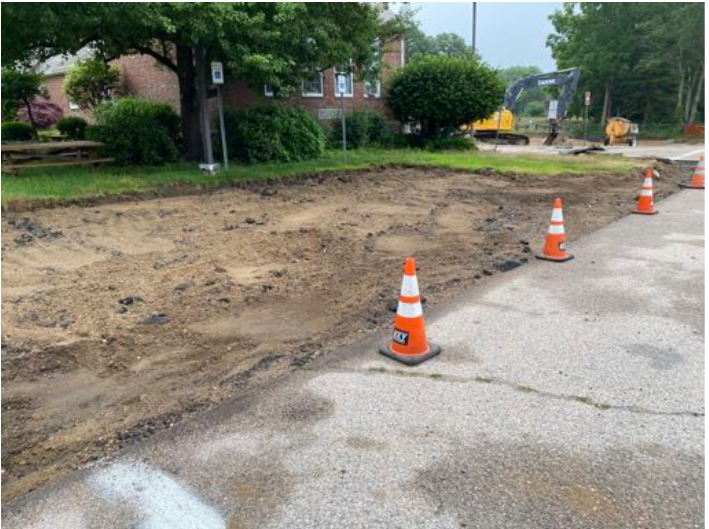
Asphalt removed at parking strip in front of school.
