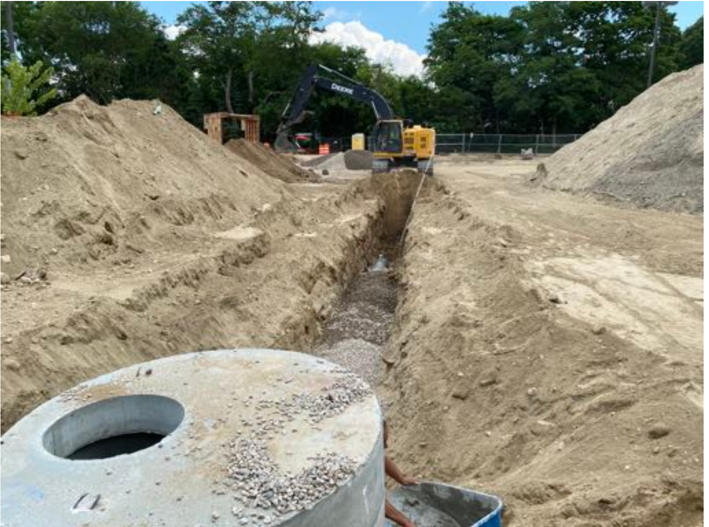
Installation of 15" pipe from DMH #5
