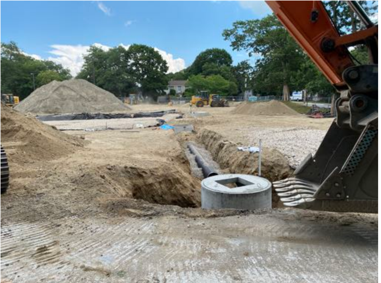
Installation of CB#1 and 12" pipe
