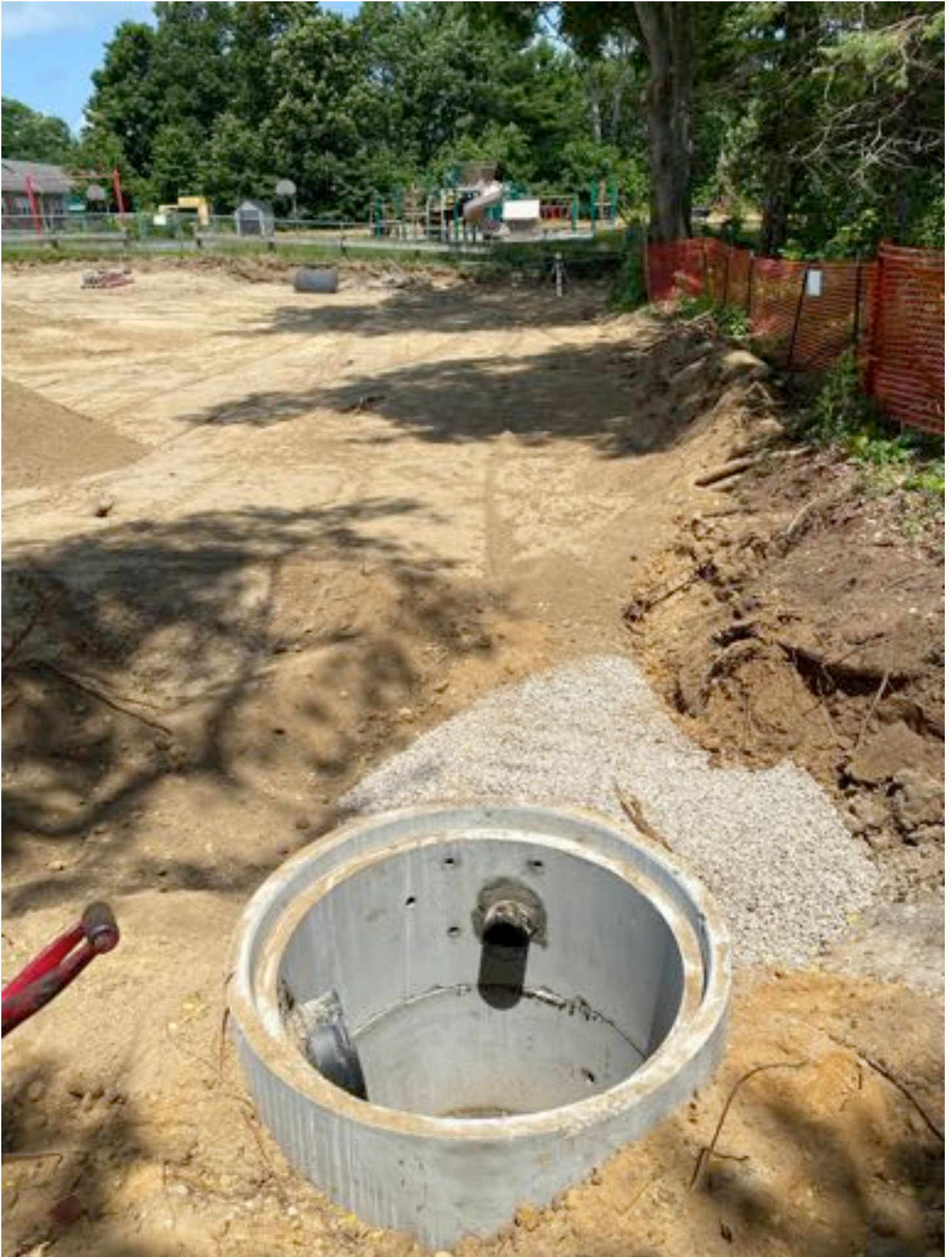
6" pipe install completed
