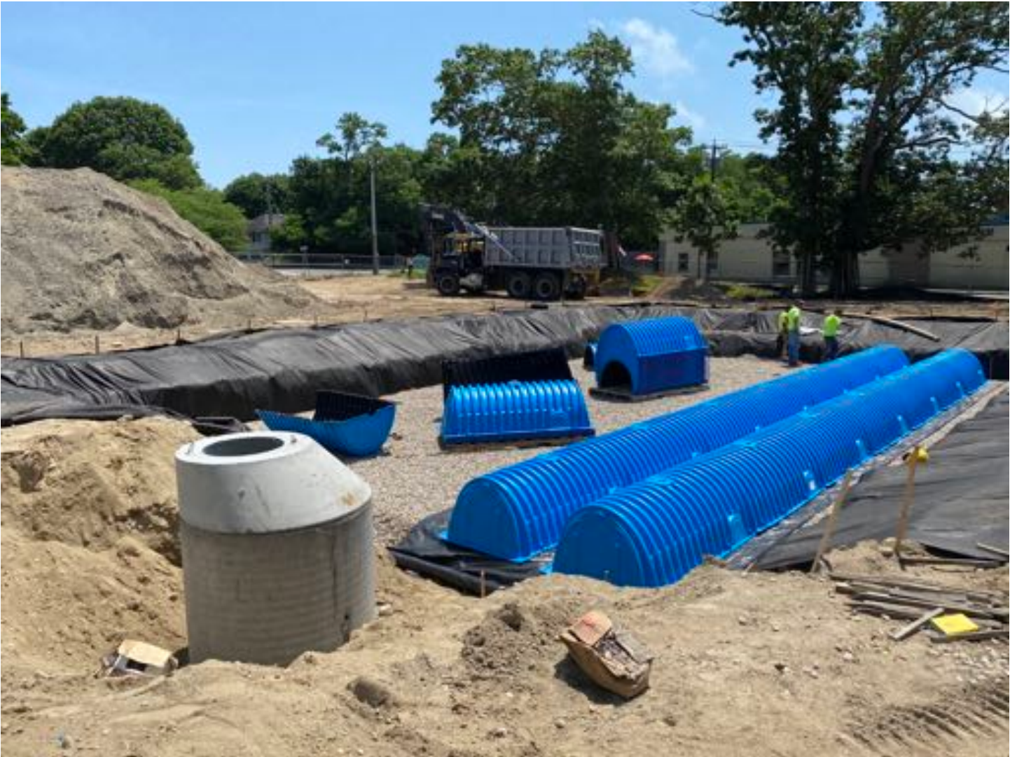
UCS #1 Stone bed complete, placement of chambers.
