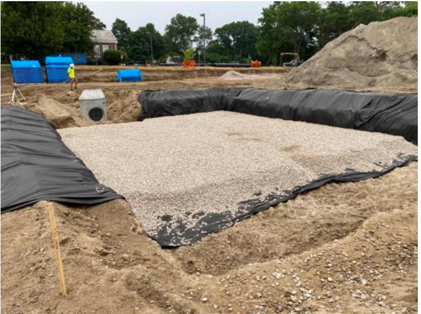
UCS #1 fabric/stone placement
