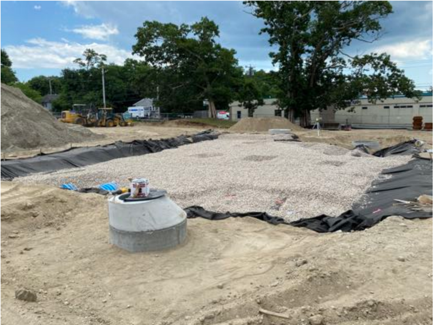
Chamber backfilling nearly complete.
