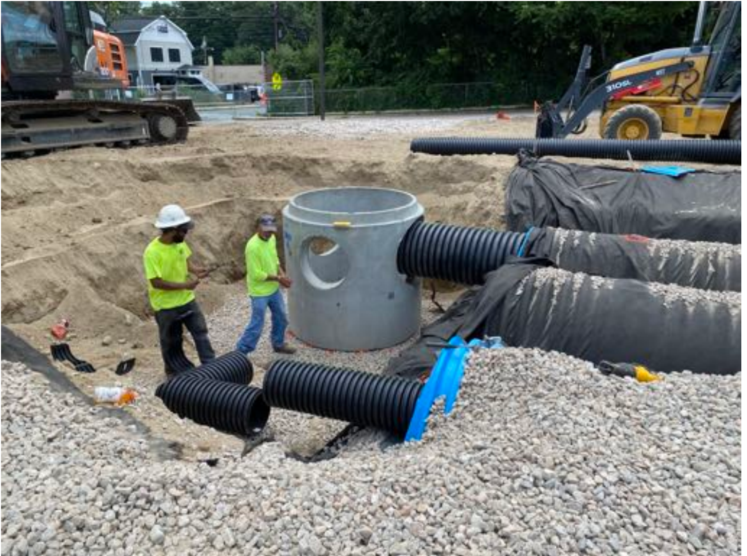
Installation of DMH2/chamber header.
