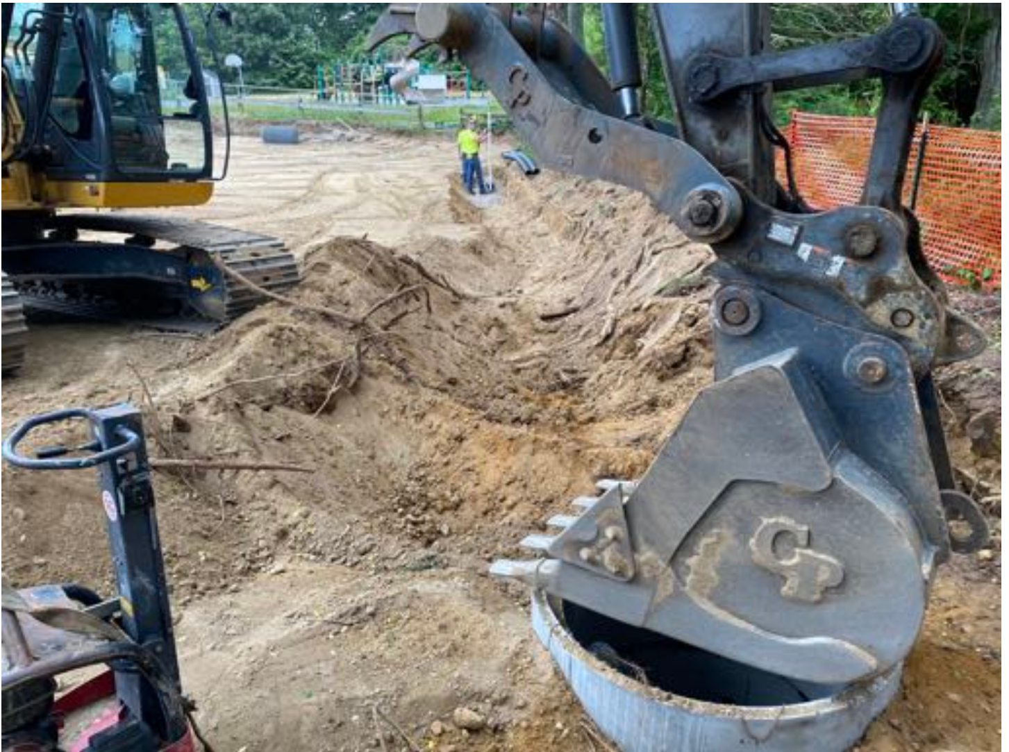
CB#8 installed, 6" pipe being installed.
