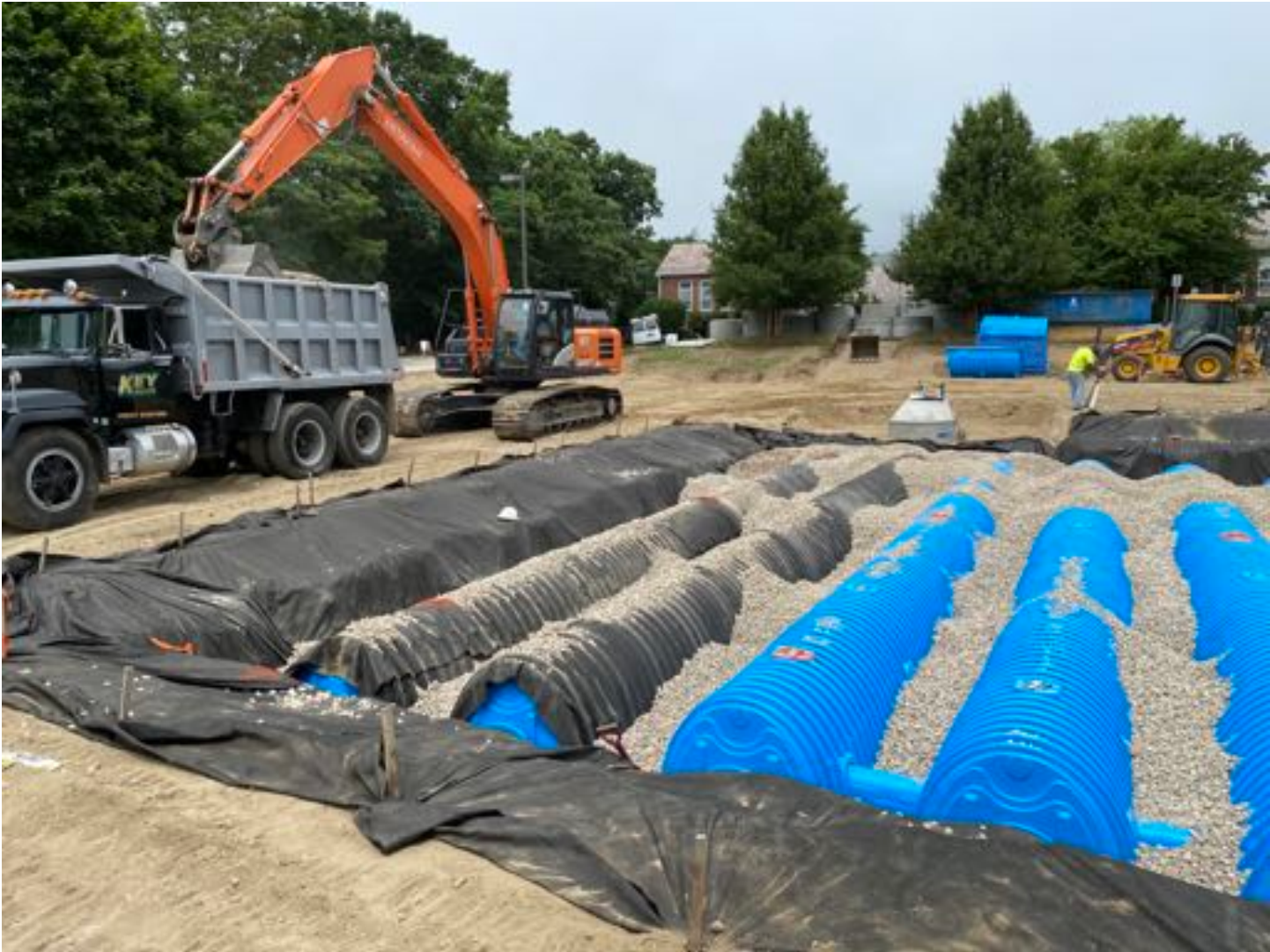
Chamber backfilling continues
