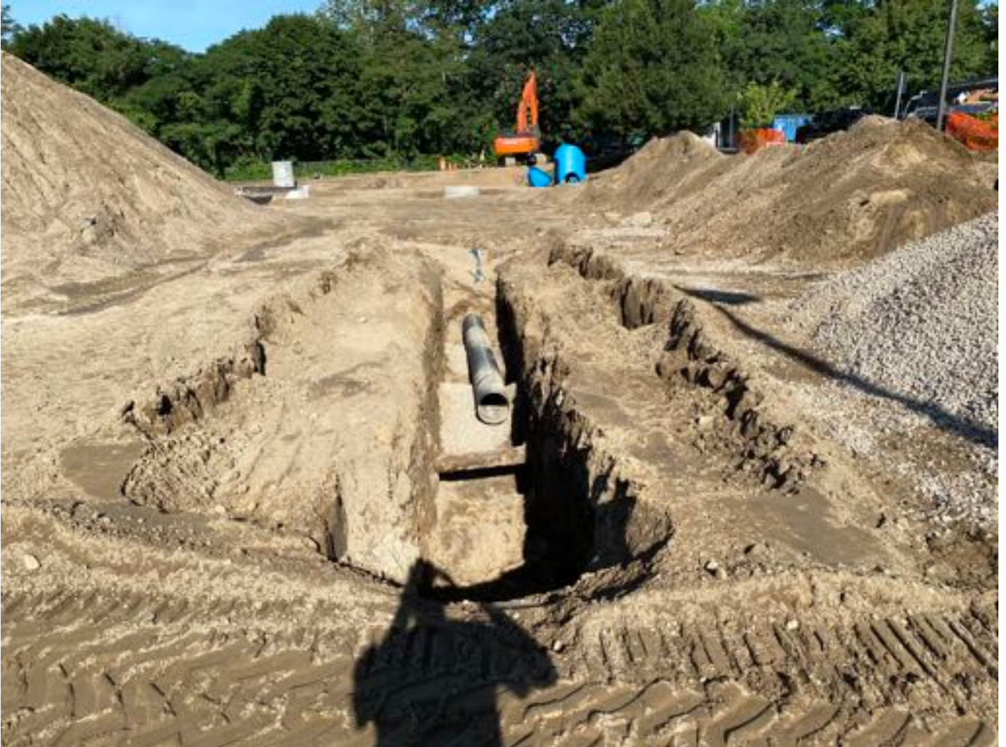
15" pipe installed to water main crossing conflict
