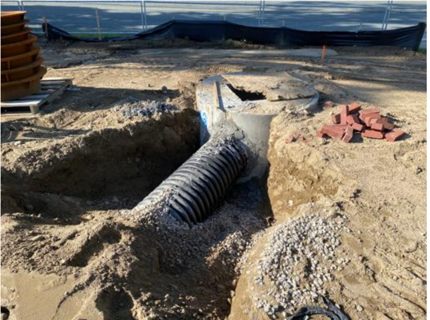
12" pipe installed to CB #2
