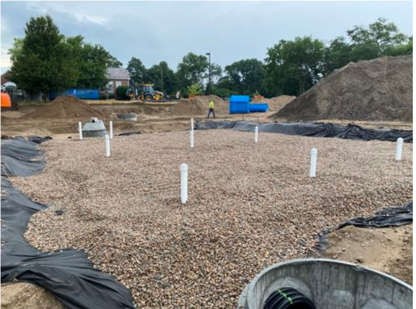
UCS #1 cleanouts installed, stone backfill complete.
