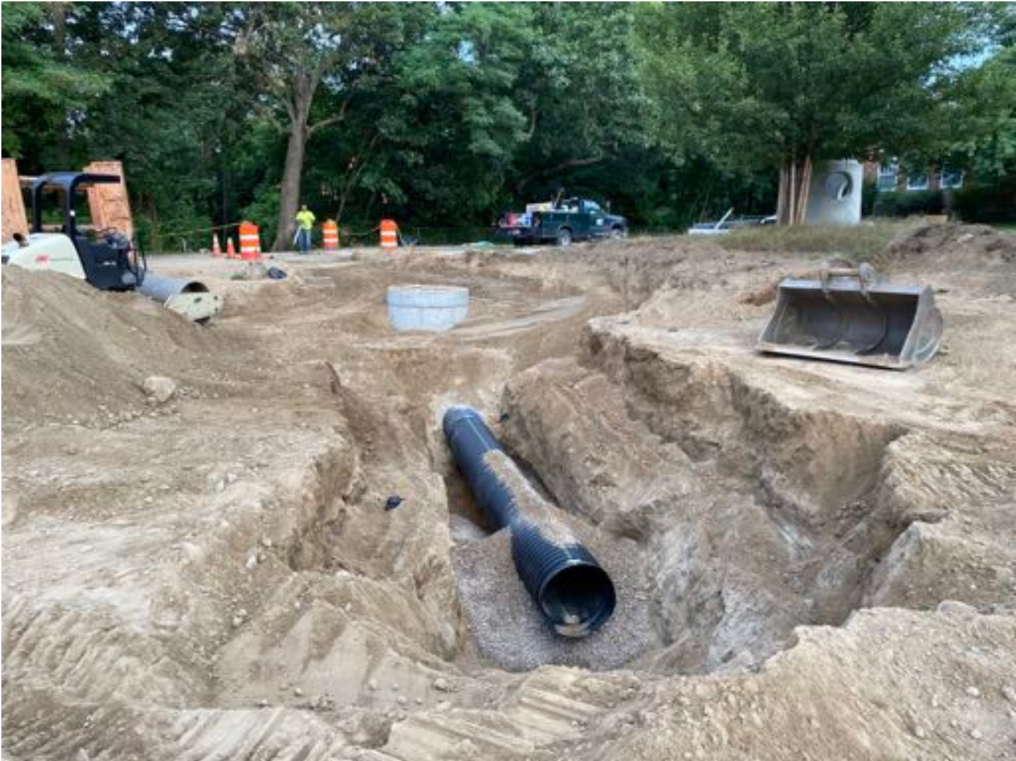
DMH #7 backfilled, 24" pipe installed.
