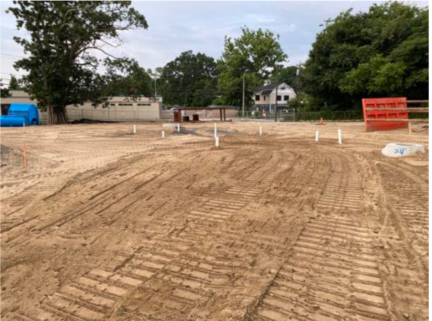
UCS #1 partially backfilled.
