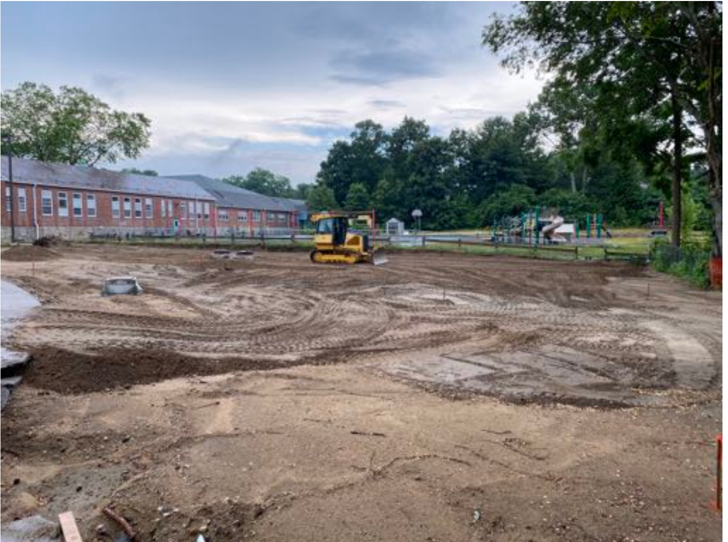
Placement of spoils in new parking area.
