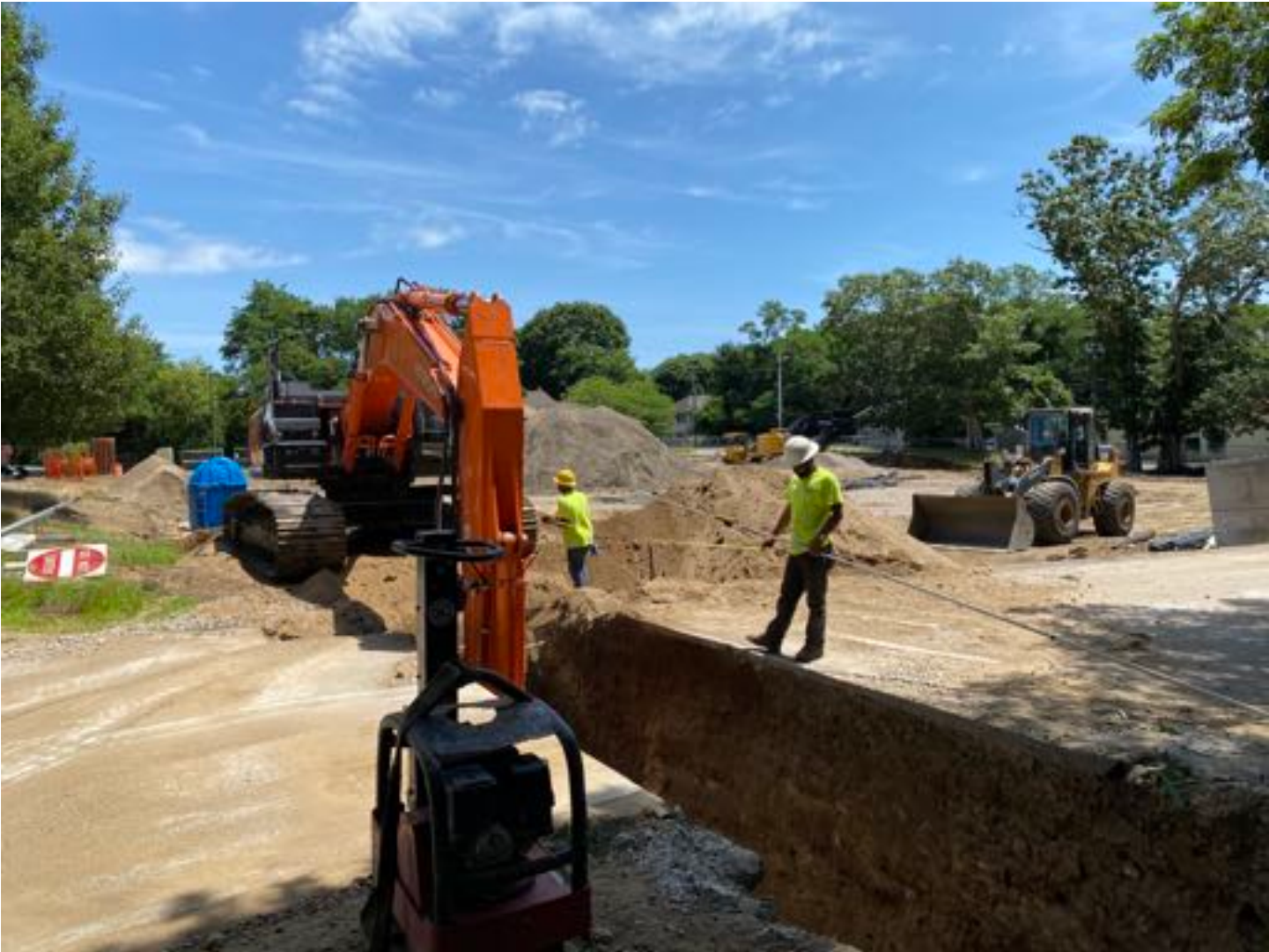
Excavation for 24" pipe
