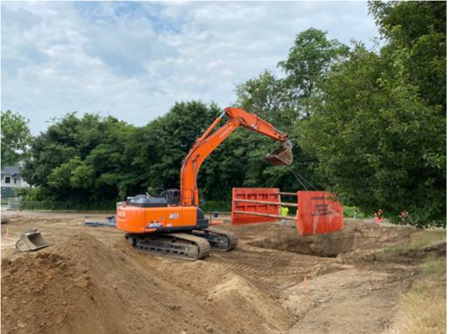
Installation of shoring for DMH #7.
