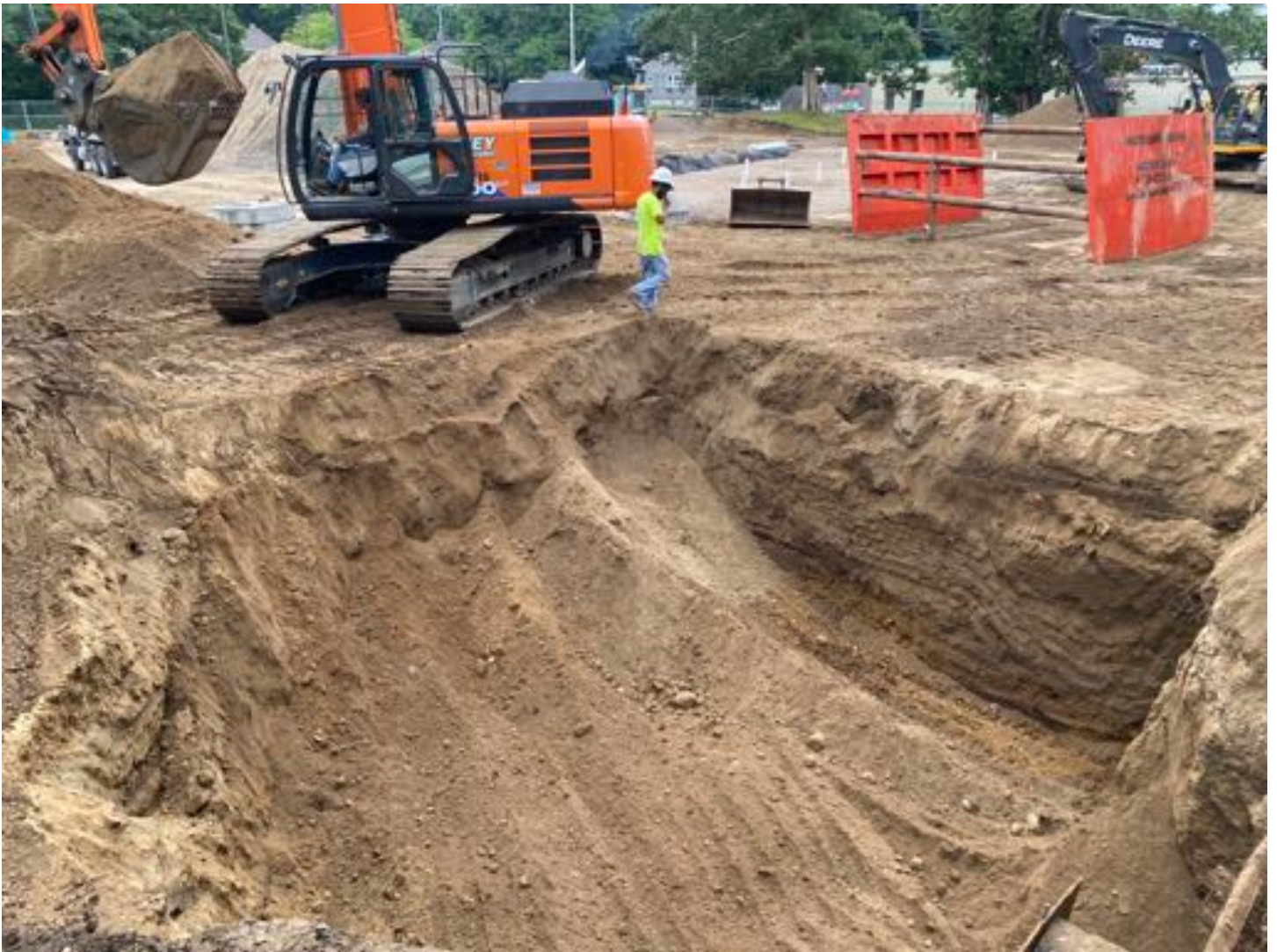
Excavation for DMH #7
