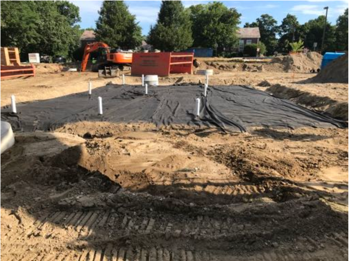
Fabric placed over UCS #1
