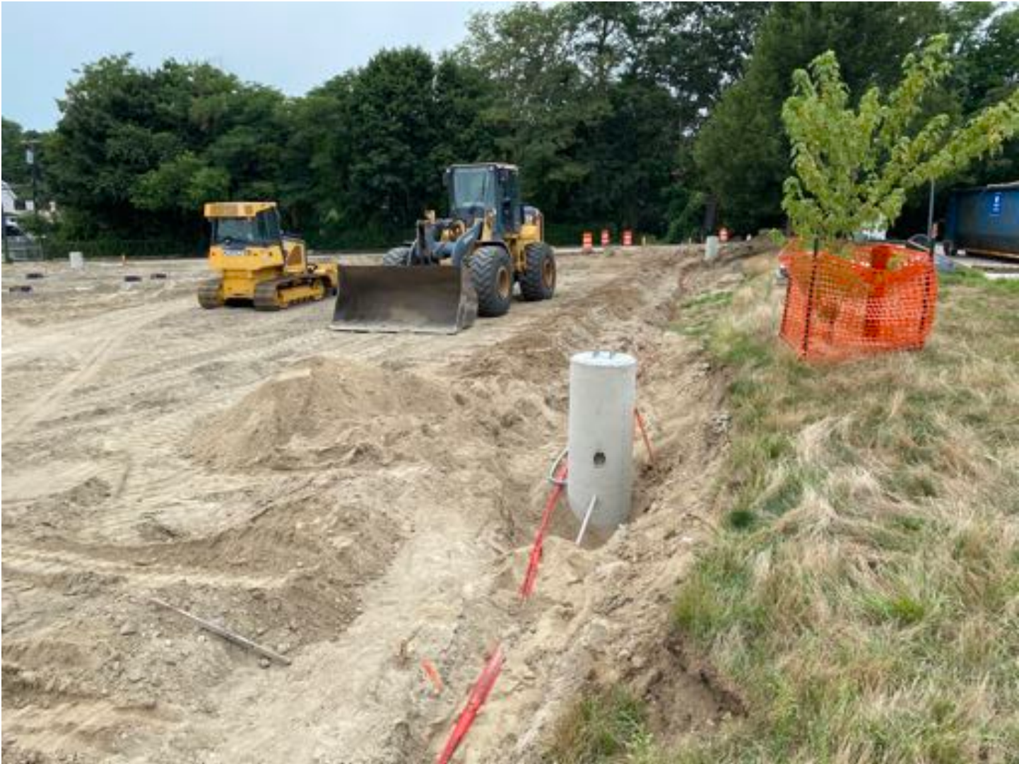
Light bases installed in main parking lot.
