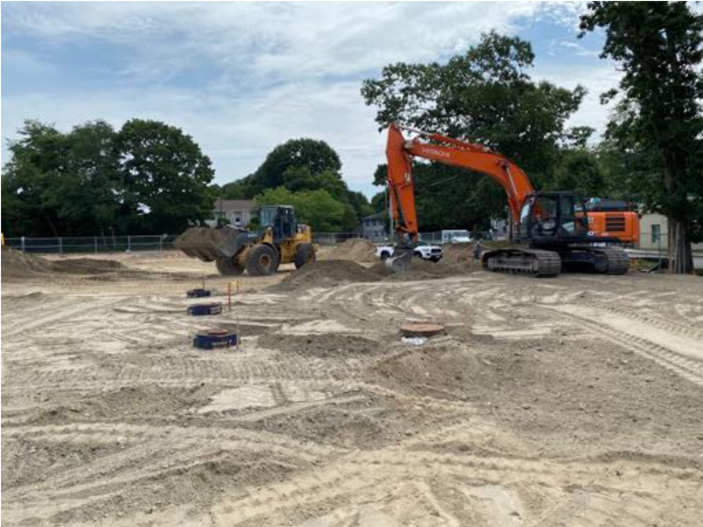
Reclaimed base being spread along south side of parking lot.
