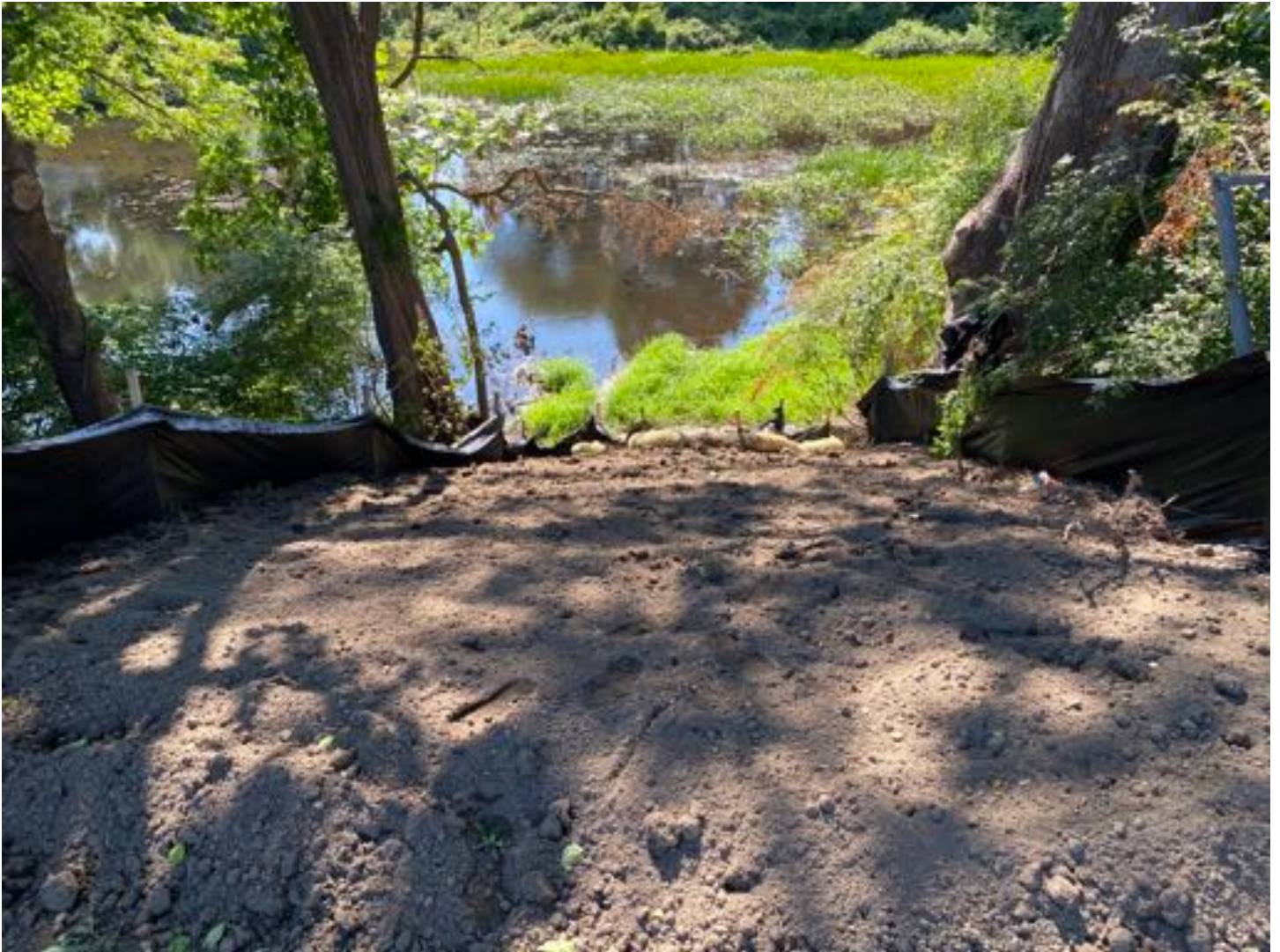
Topsoil placed on slope of 24" pipe outfall.
