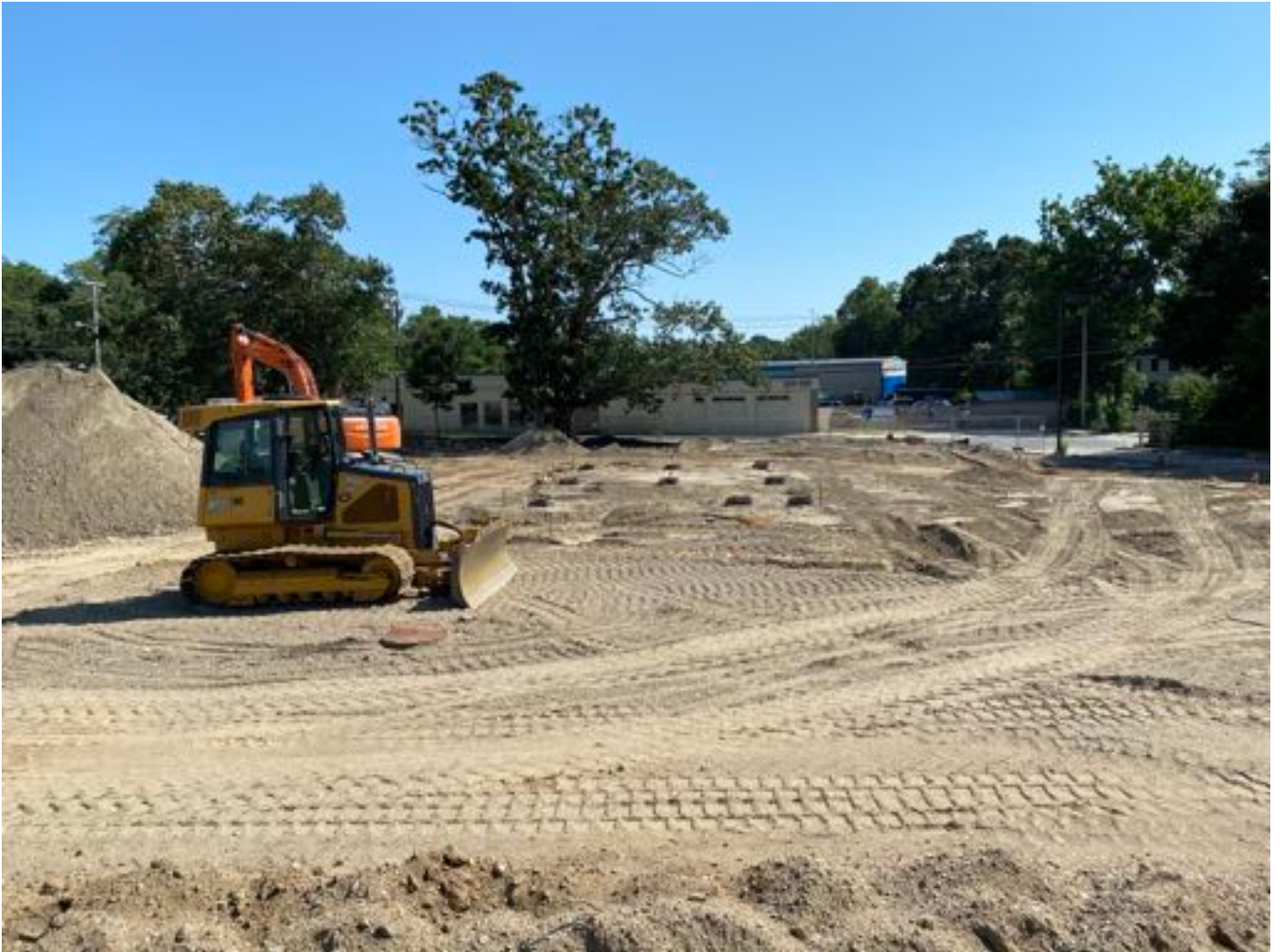
Placement of reclaimed base in main parking area.
