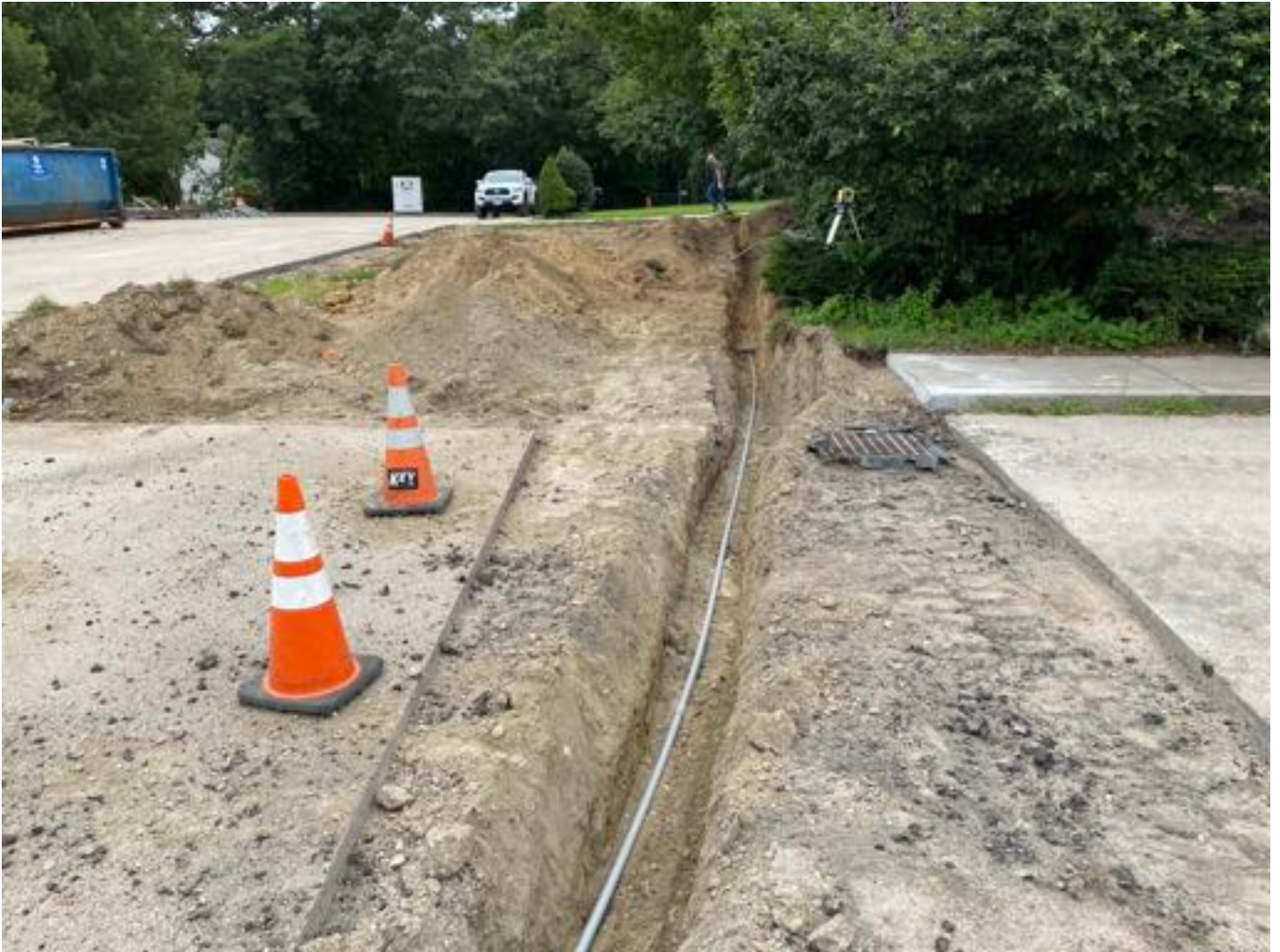
Conduit installed in front of building.
