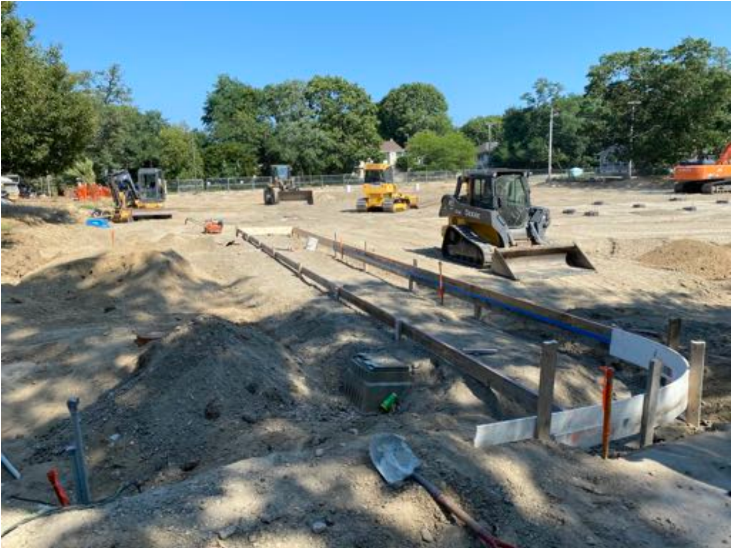
5' wide monolithic sidewalk/curb formed.
