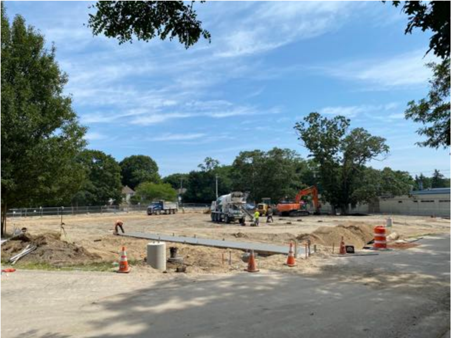
Placement of concrete for sidewalk/cleanouts.
