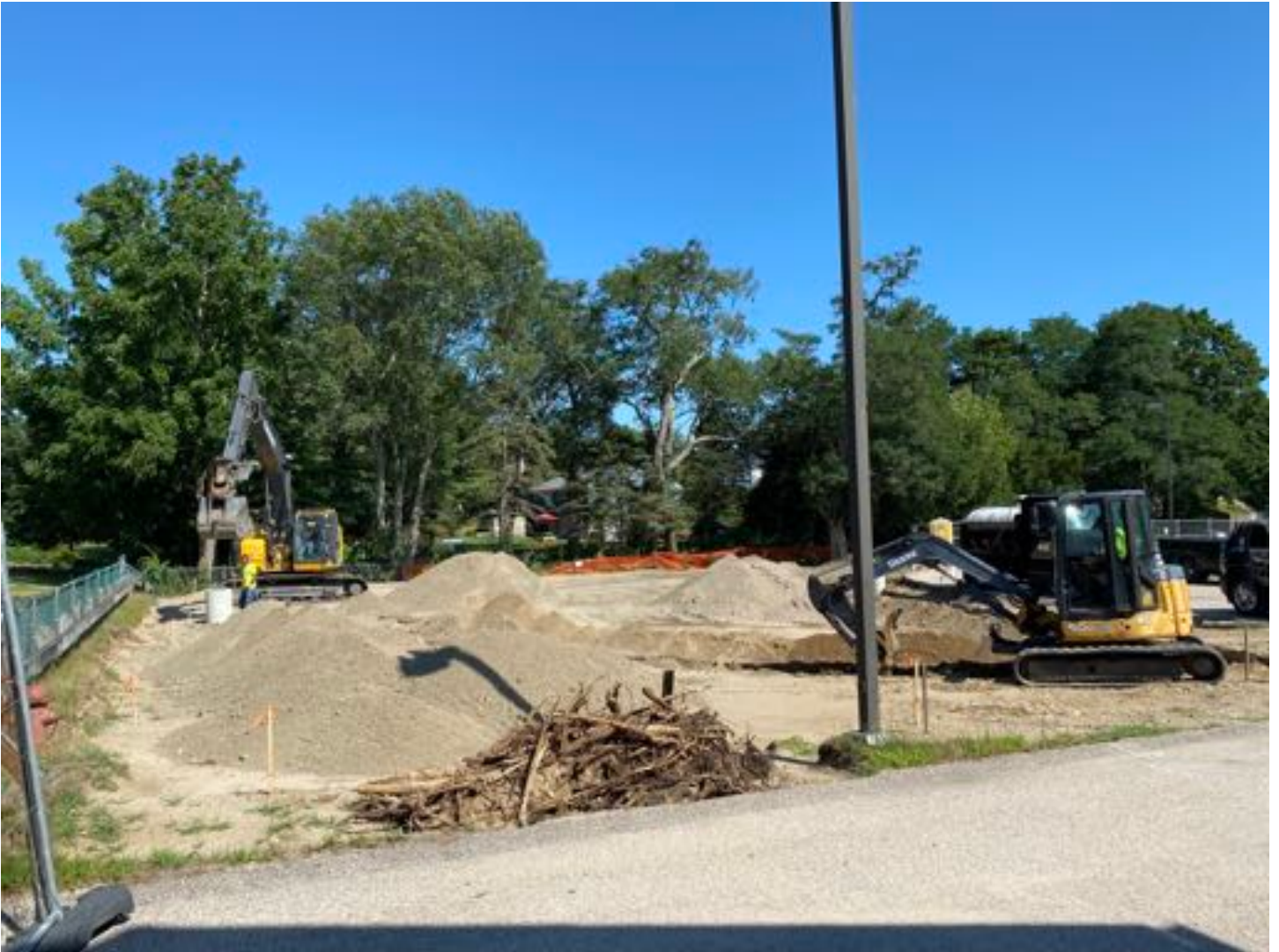
Electrical conduit excavation/placement of light base in parking lot addition.
