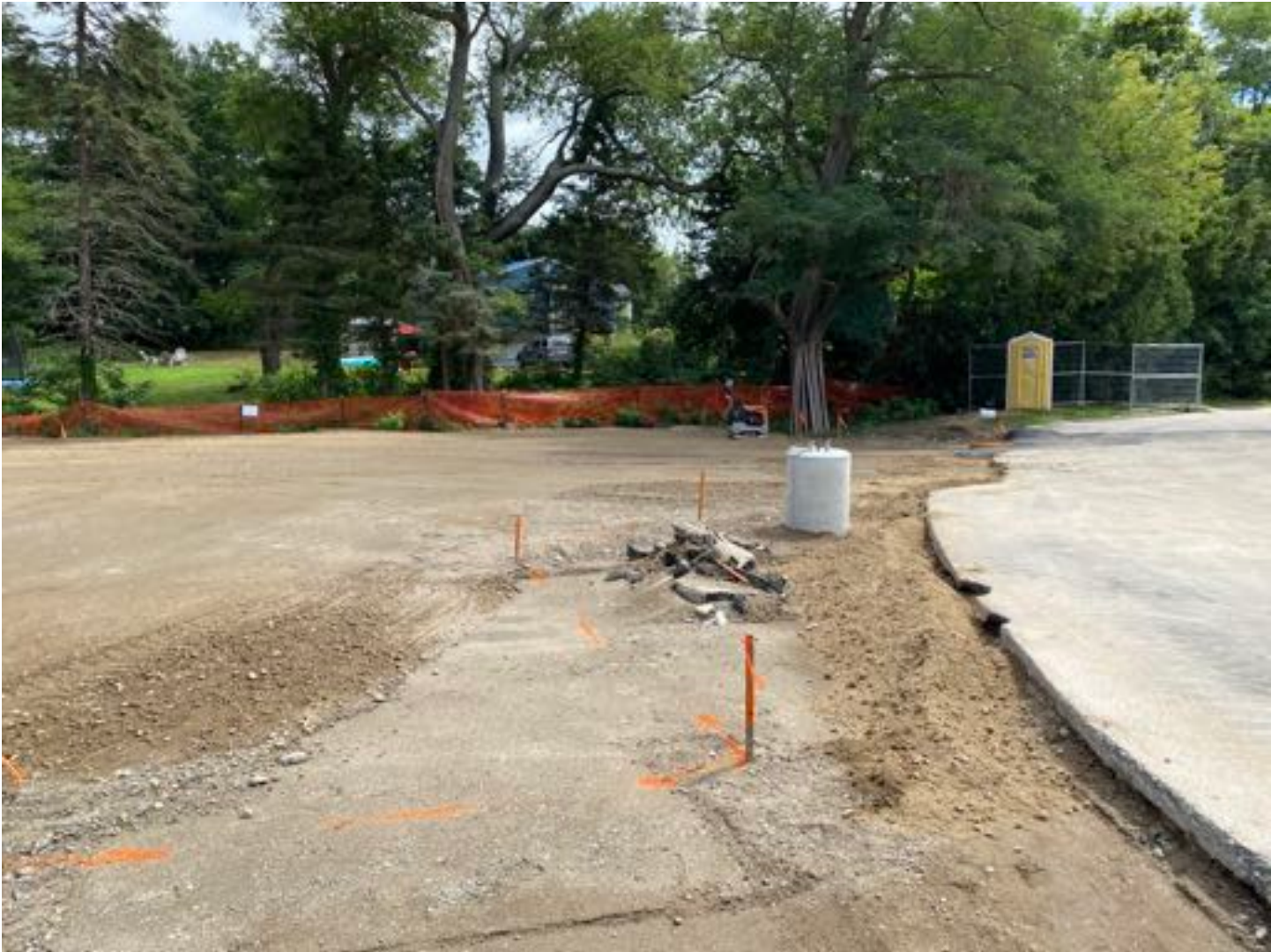
Expanded parking area graded, Prep for new curb.
