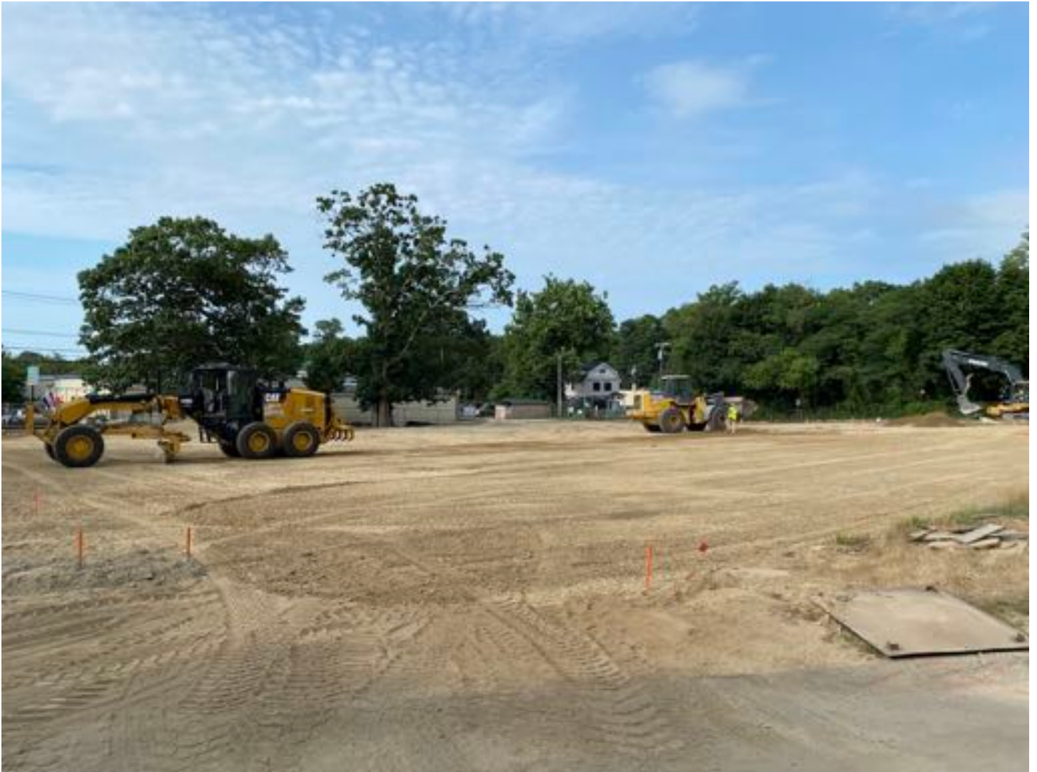
Fine grading of main parking lot.
