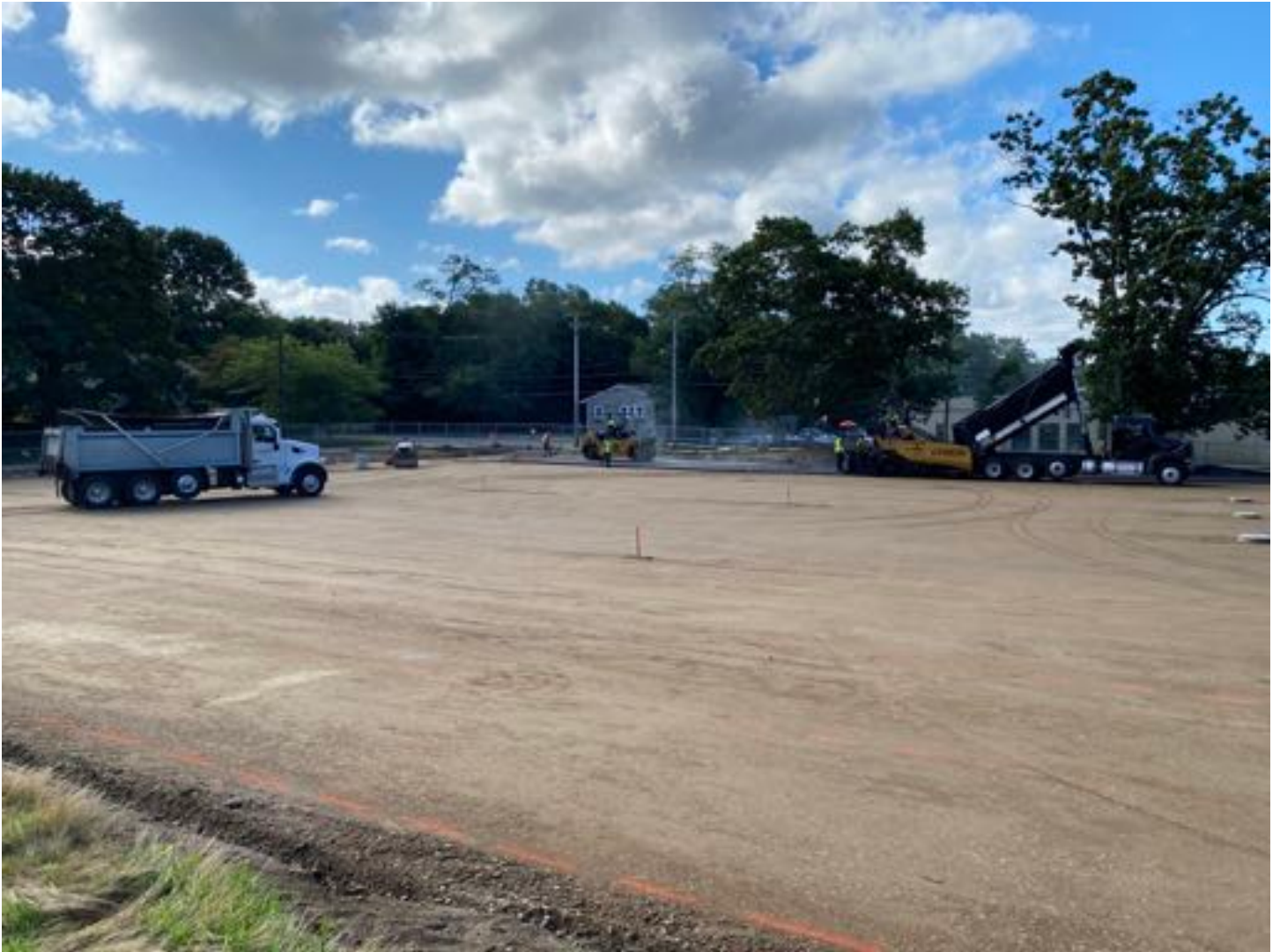
Binder placement in main parking lot.
