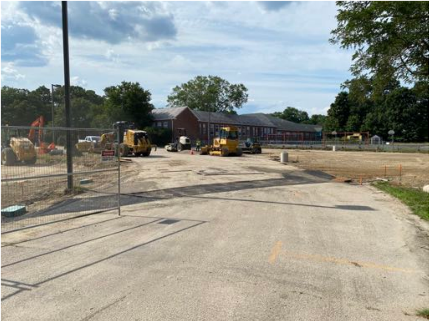
Asphalt patch at 18" pipe crossing.
