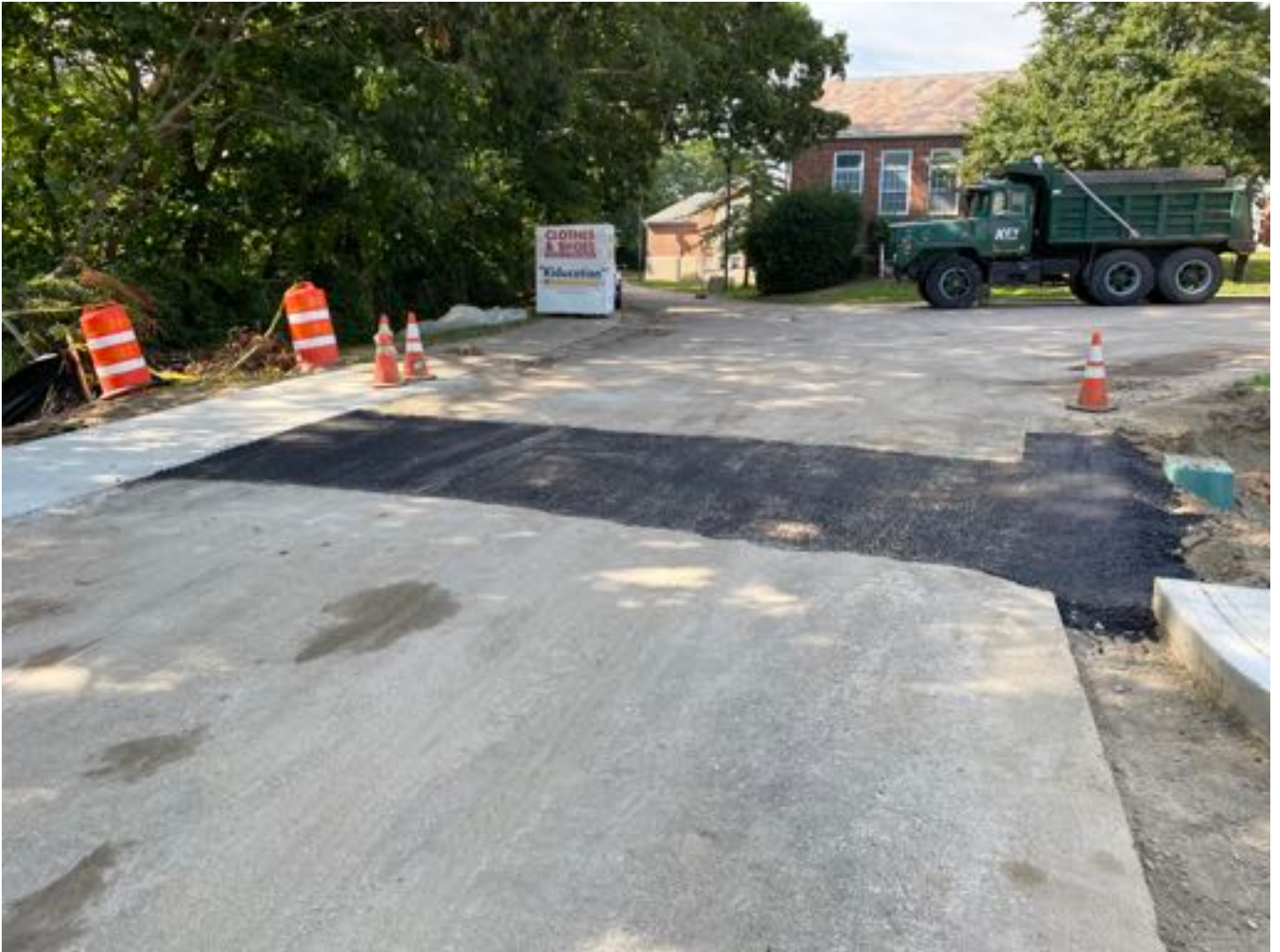
Asphalt patch/sidewalk repair at 24" pipe.
