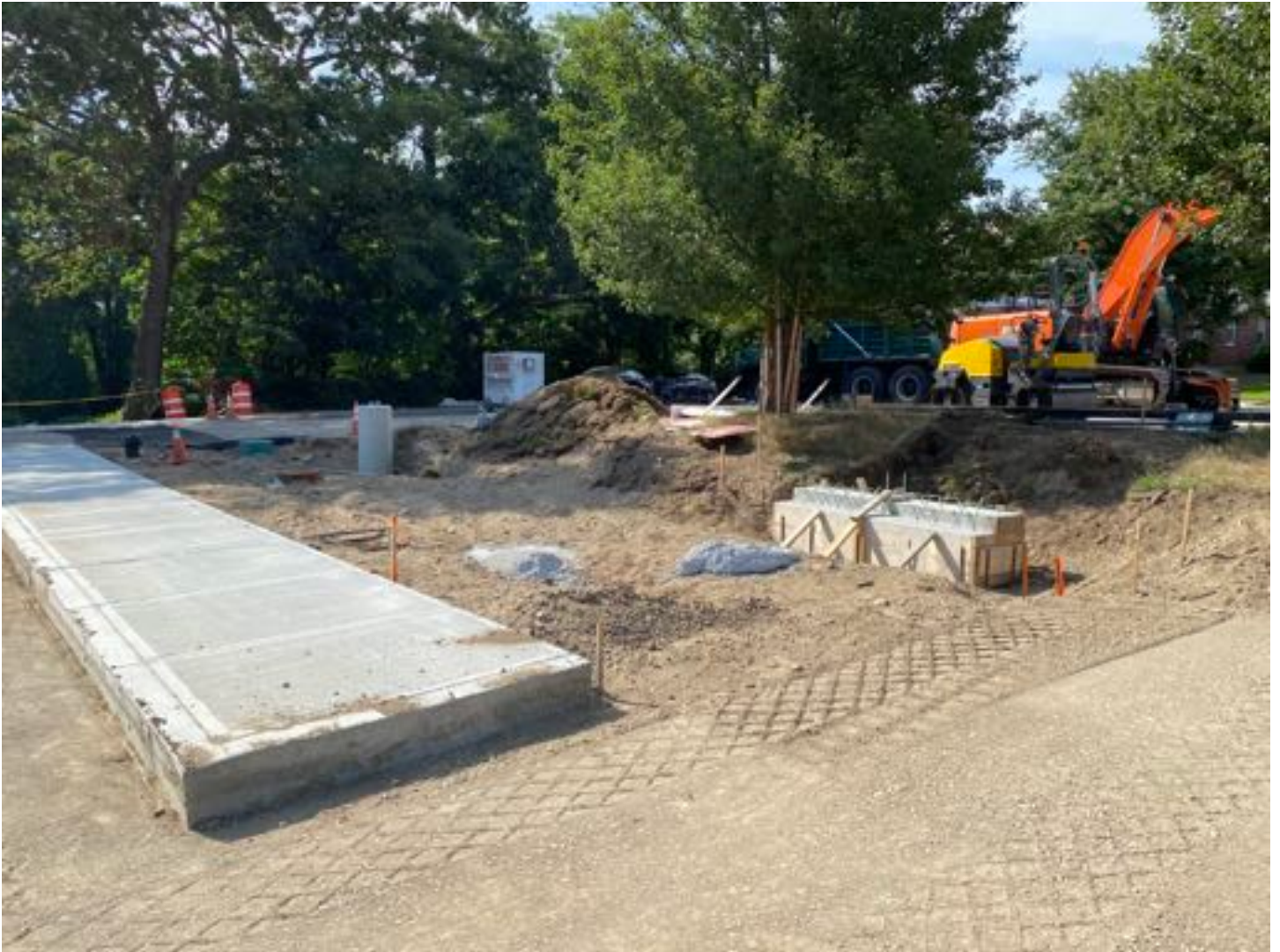
Sidewalk poured/stripped, stair footings poured.
