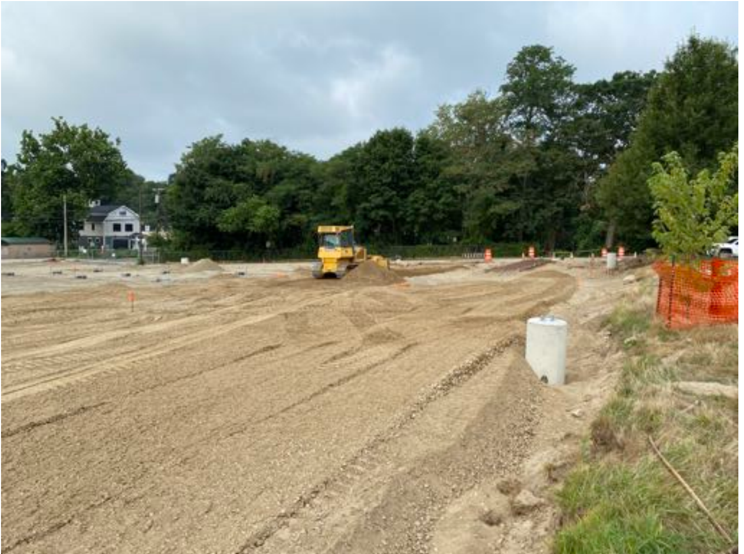
Gravel base being placed.
