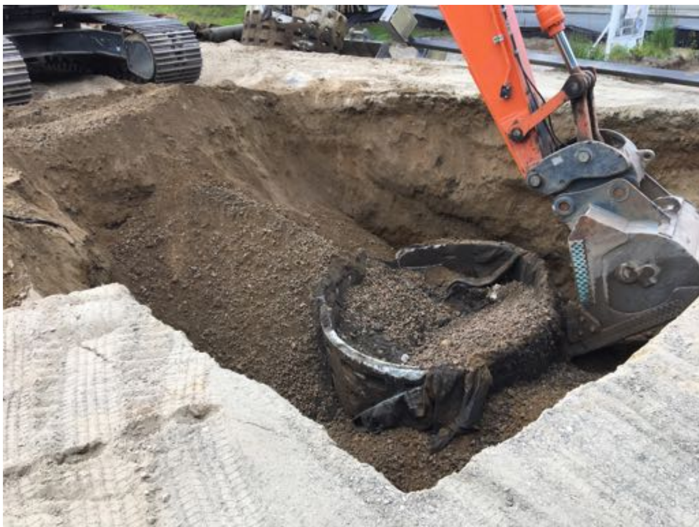
Removal of drywell (RFI #4).
