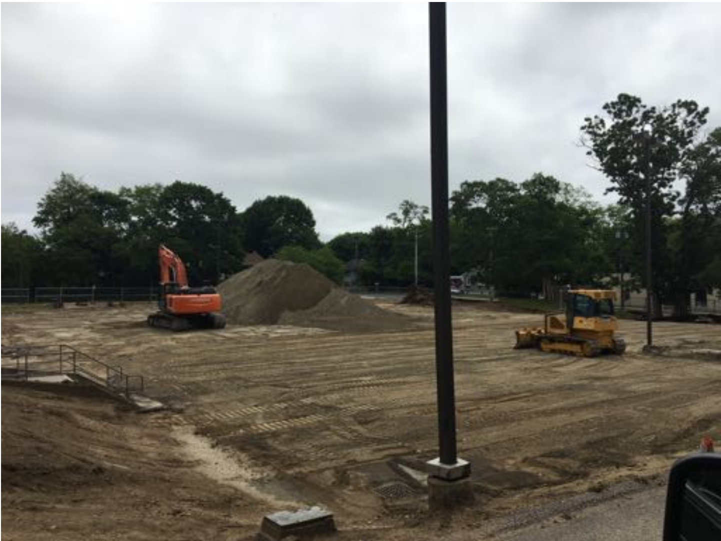
Stripping/stockpiling of Reclaim material.
