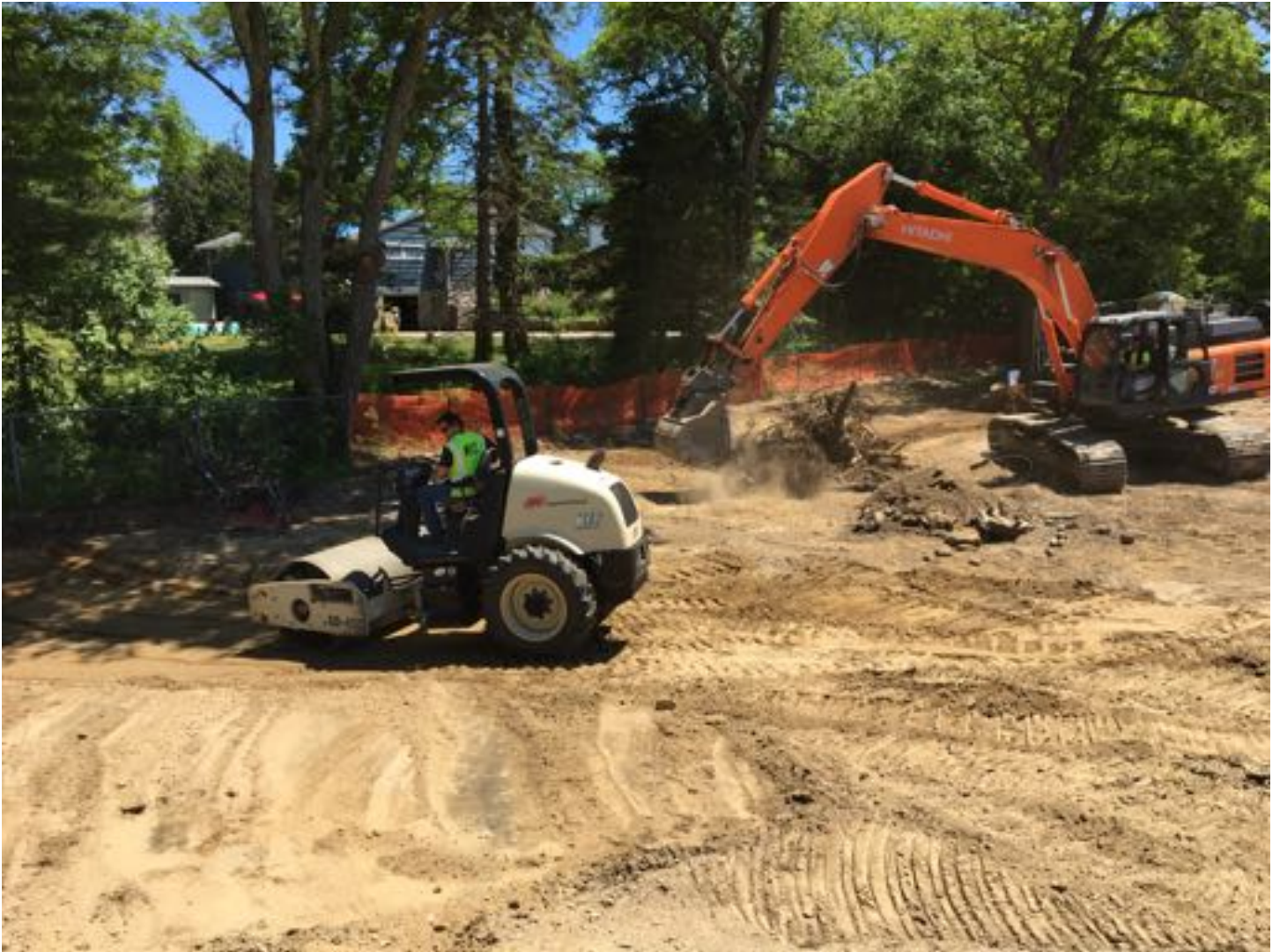
Removal of catch basin structures in former labyrinth area.
